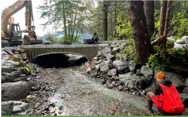
Katie Russell inspects a fish passage bridge project that improves salmon habitat in Juneau, Alaska.
