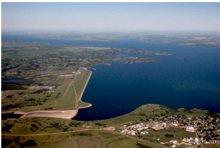
Aerial view of Garrison Dam, impounding Lake Sakakawea on the Missouri River (photo courtesy of USACE).
