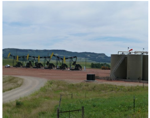
Eco-pad with 6 pumping units in Dunn County, North Dakota. Horizontal drilling in different directions has made it possible to have multiple pumping units spaced close together on a single large well pad (photo courtesy of NRCS).
