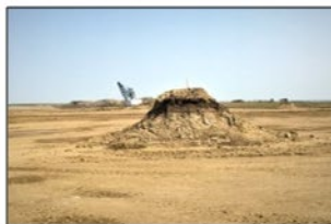
Topsoil and subsoil are removed and respread in two separate lifts.
