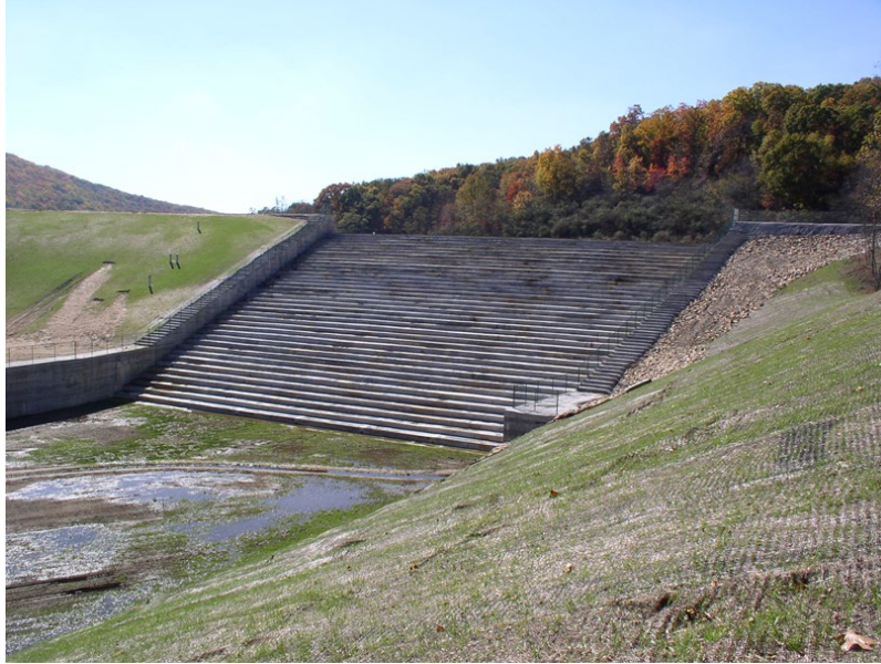
Figure 2 - Example of a Roller-Compacted Concrete Auxiliary Spillway
