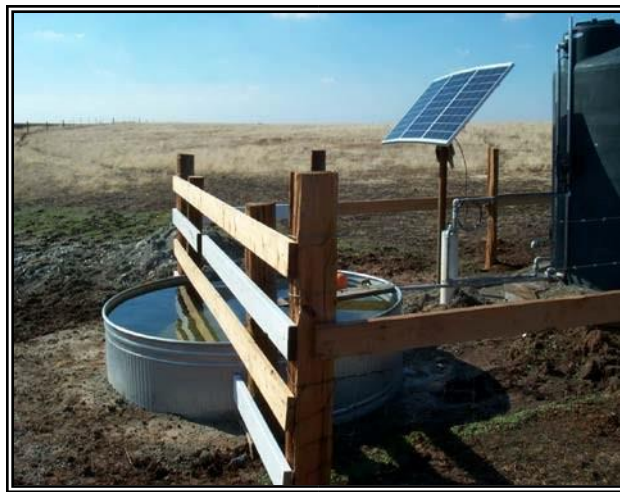
Figure 5.1 – PV solar array with storage tank and stock. (Source: “Renewable Energy Primer-Solar.”)
