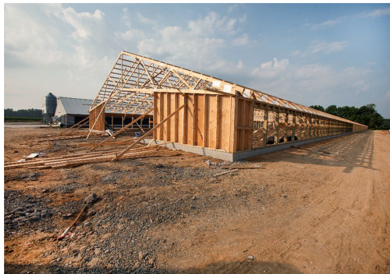
Poultry house under construction.
