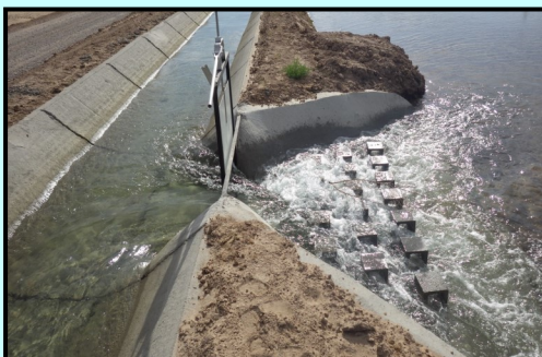
High-flow turnout in action Las Cruces, NM
