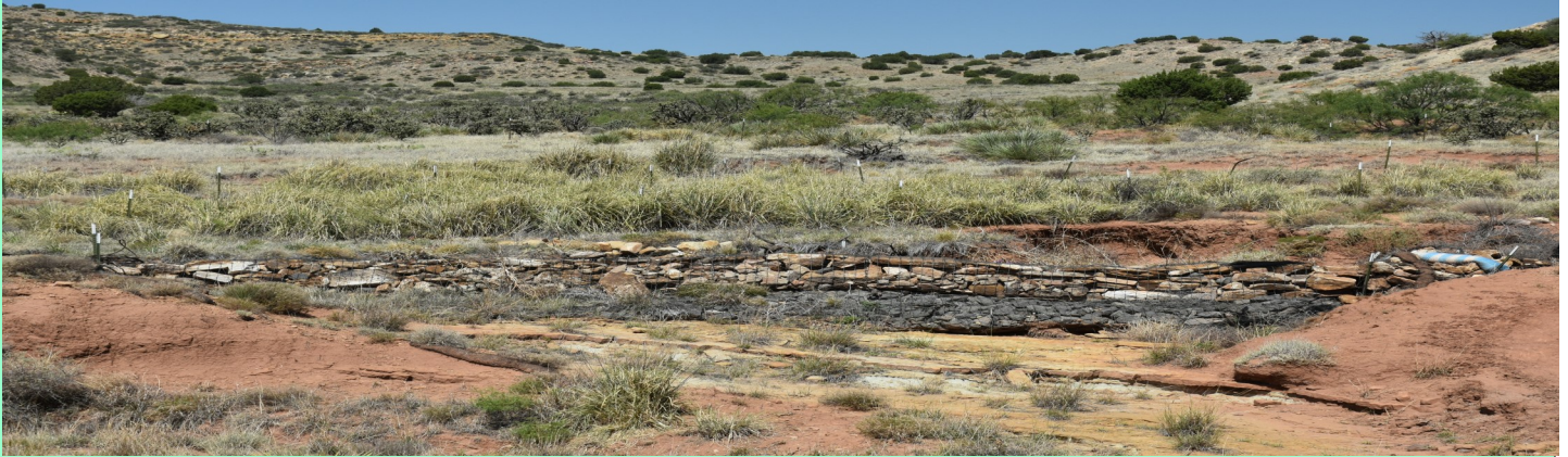
Rock and brush structure for erosion control in a gully.
