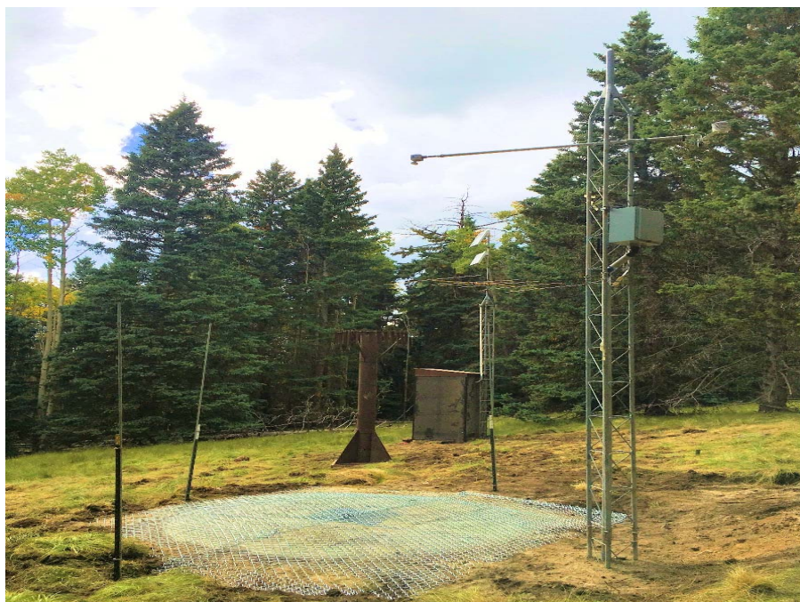
The newly constructed La Garita Hill SNOTEL site.
