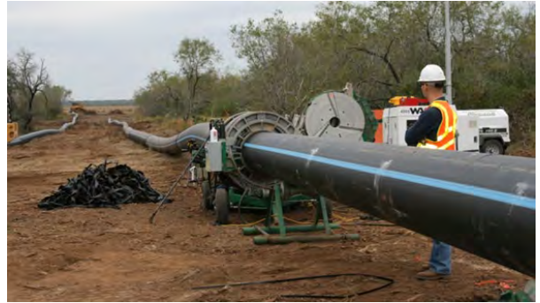
Fusion Welding HDPE Pipe
