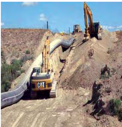
Placing HDPE Pipe in Trench
