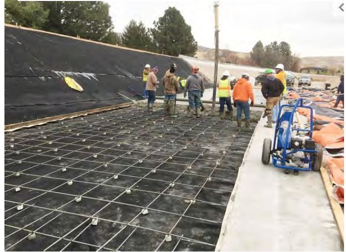
Pouring Concrete Slab Over Composite Liner
