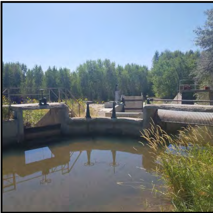
Diversion structure at northern end of canal
