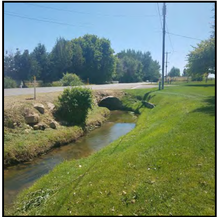
Existing conditions in residential areas
