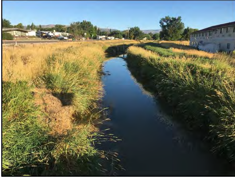
Photo 5: A trail would be constructed along the Steinaker Service Canal as part of the Proposed Project. Vegetation along the alignment of Steinaker Service Canal included: reed canarygrass, Canada thistle ( Cirsium arvense ), smooth brome ( Bromus inermis ), sunflower ( Helianthus sp.), alfalfa ( Medicago sativa ), crested wheatgrass ( Agropyron cristatum ), scouring rush, perennial ryegrass ( Lolium perenne ), prickly lettuce ( Lactuca serriola ), Indian ricegrass ( Achnatherum hymenoides ), milkweed ( Asclepias speciosa ), groundsel ( Senecio vulgaris ), and curlycup gumweed.
