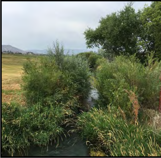
Representative conditions along Ashley Canal segment surveyed.
