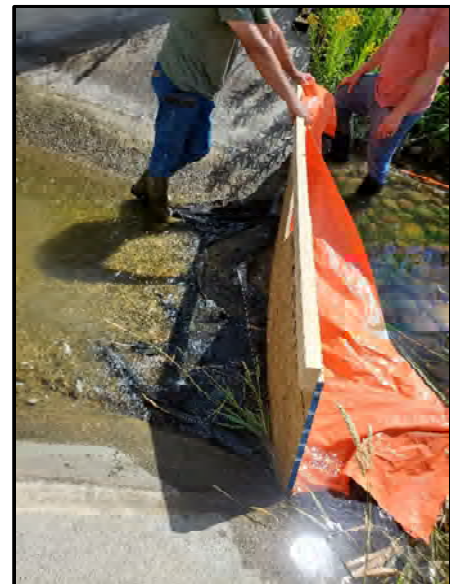
Figure 1 - Attempt to measure discharge using a V-notch weir
