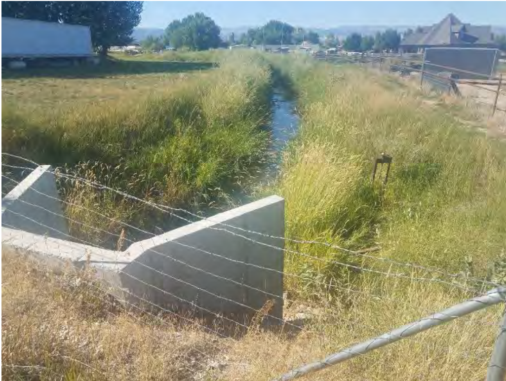
16 – Site Conditions | North
