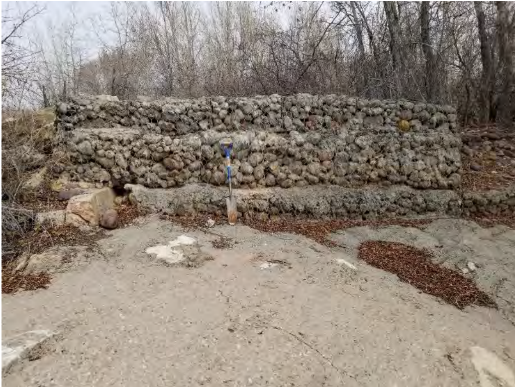
03 – Site Conditions | Northwest
