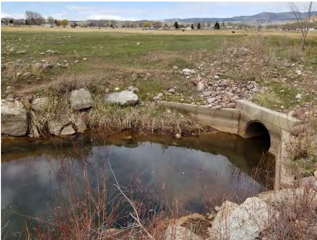
03b – Site Conditions | West
