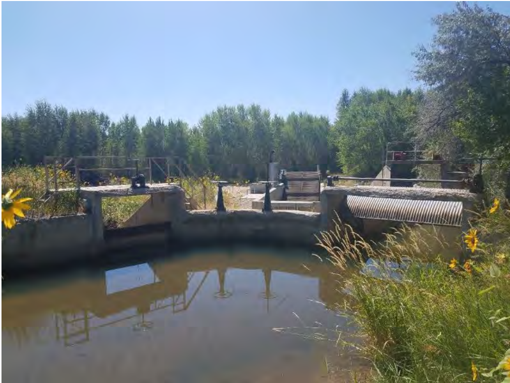
01 – Site Conditions | South
