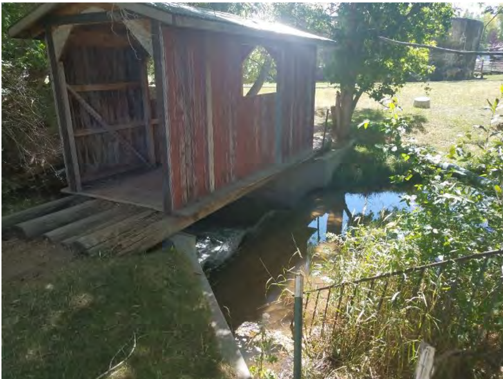
07 – Site Conditions | Southeast
