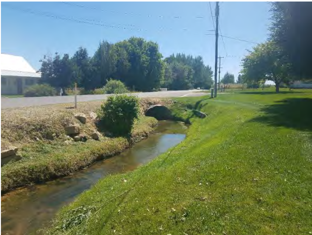
05 – Site Conditions | Southeast
