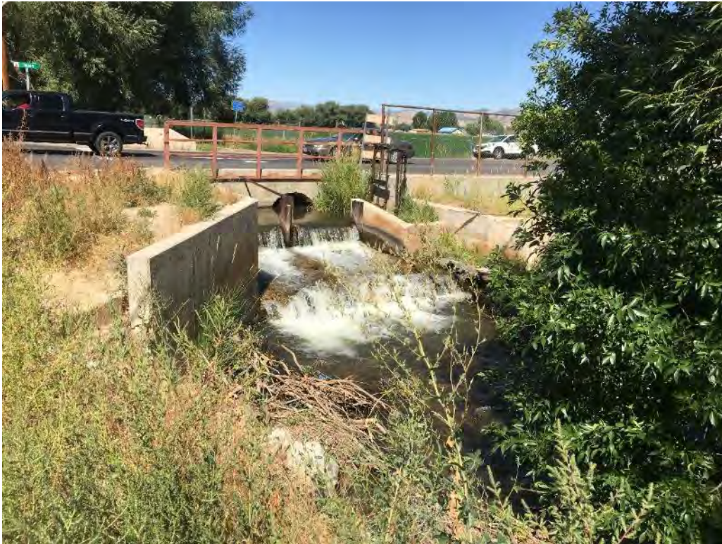
10 – Site Conditions | North
