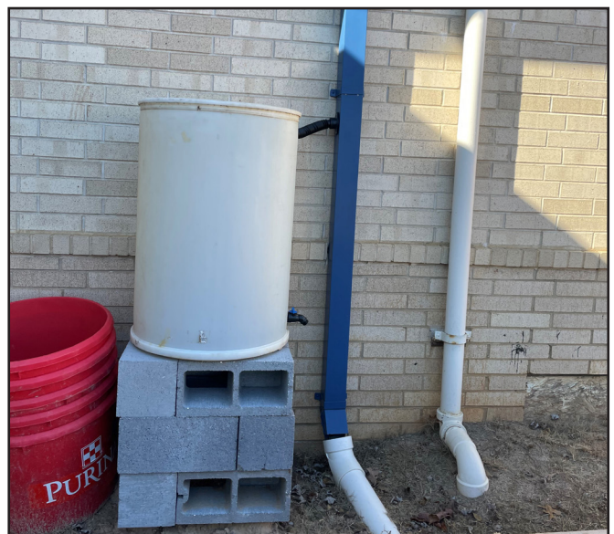
Rain barrel collecting rain water for irrigation
