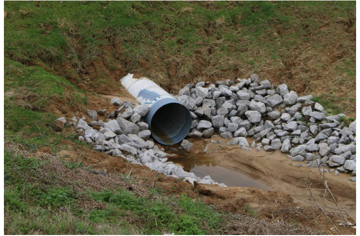
Part of Sledge Taylor’s grade stabilization Structure
