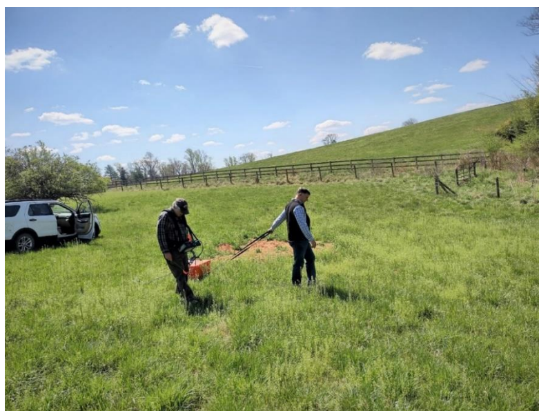
Figure 1. Alan Moore (GPR operator) and Dr. Bender (Professor of Engineering) operating the GPR in search of a ductile water line.
