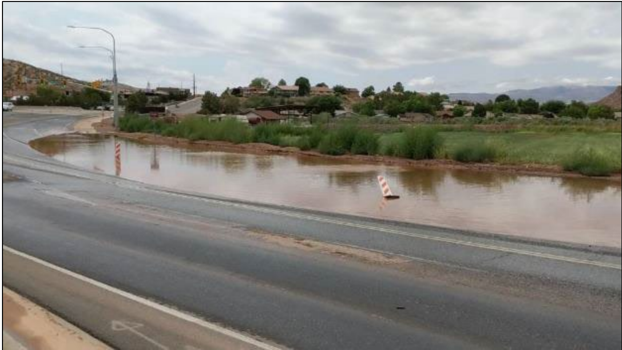
Figure 2-10. Warner Valley Disposal Pipeline Flooding (Looking at flooding along River Road near the disposal pipeline outlet at Fort Pearce Wash)
