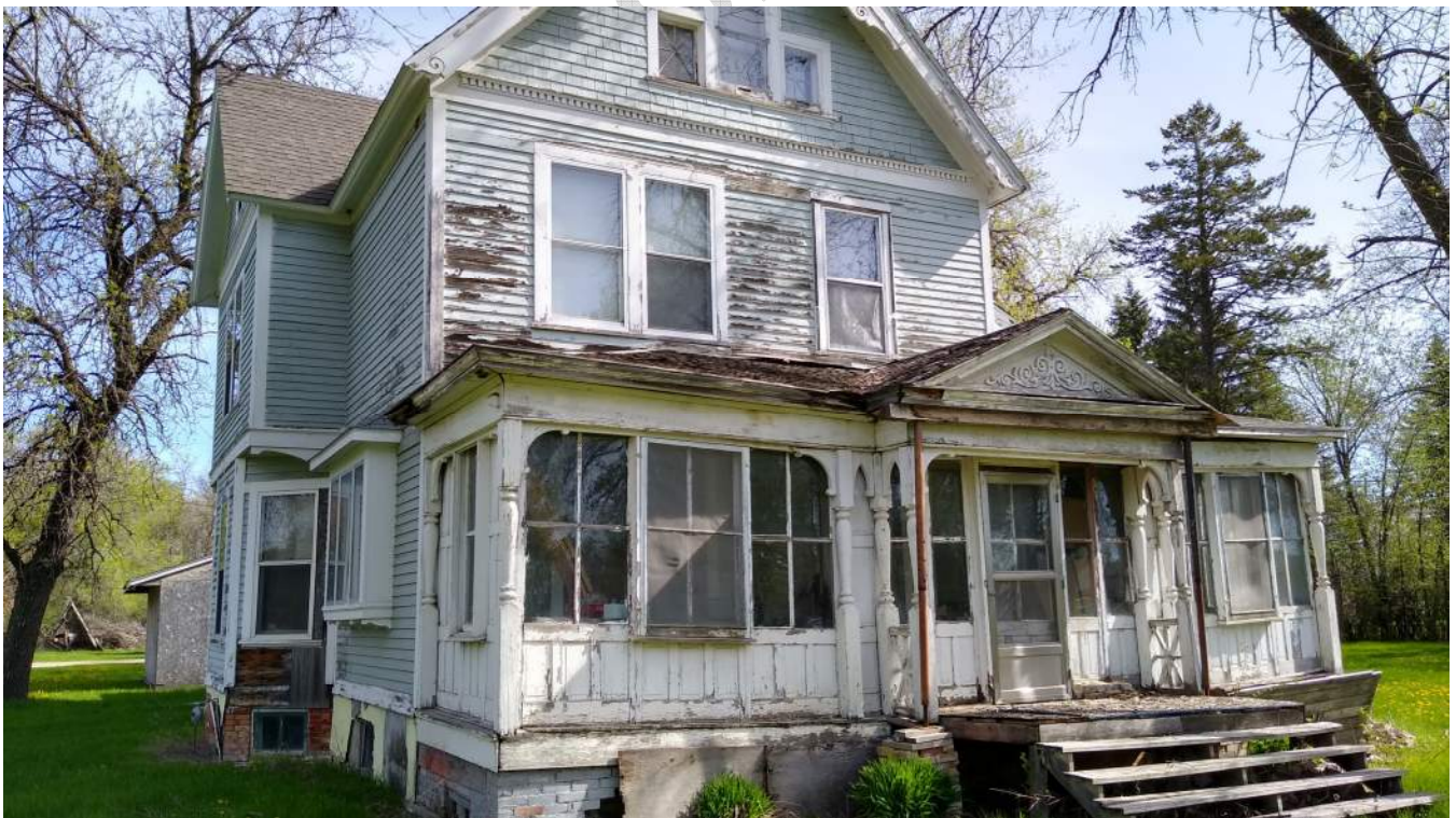
32CS5120 South West Oblique facing Northeast
