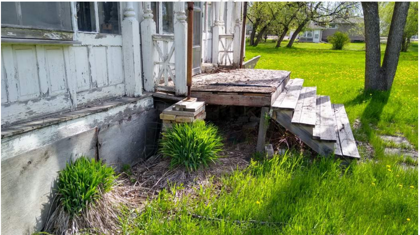
32CS5120 Porch Brick Removal
