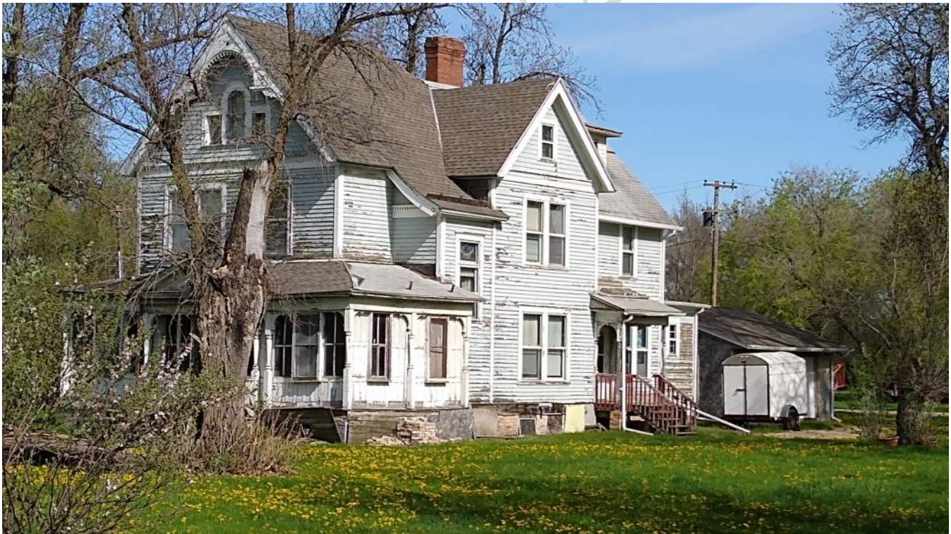
Figure 8: 32CS5120 Oblique facing Northwest. 47.006476, - 97.220032
