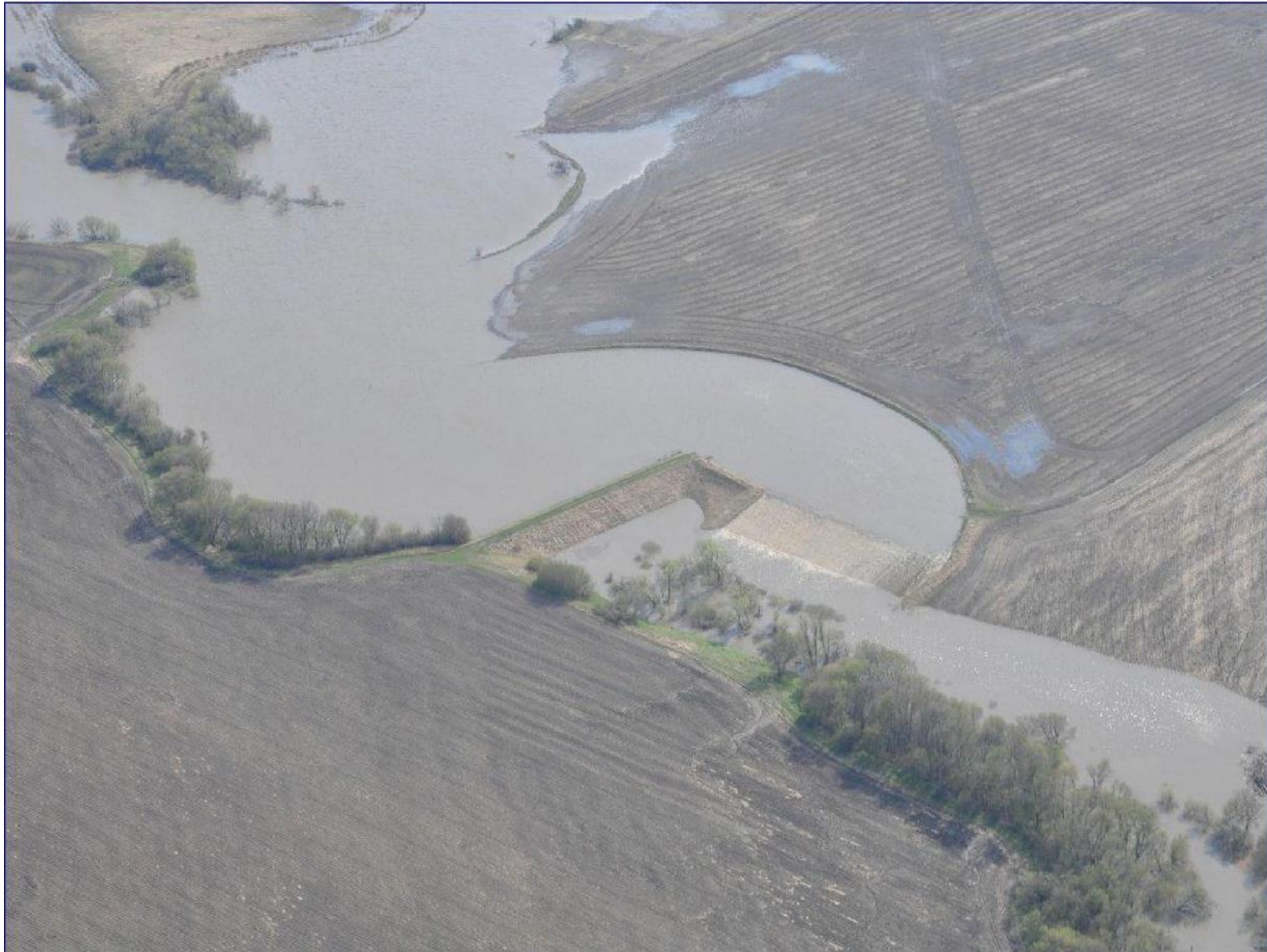
Figure 3.3.2h: 2013 Historic Event Areal Imagery for Morrison Dam Looking Southwest
