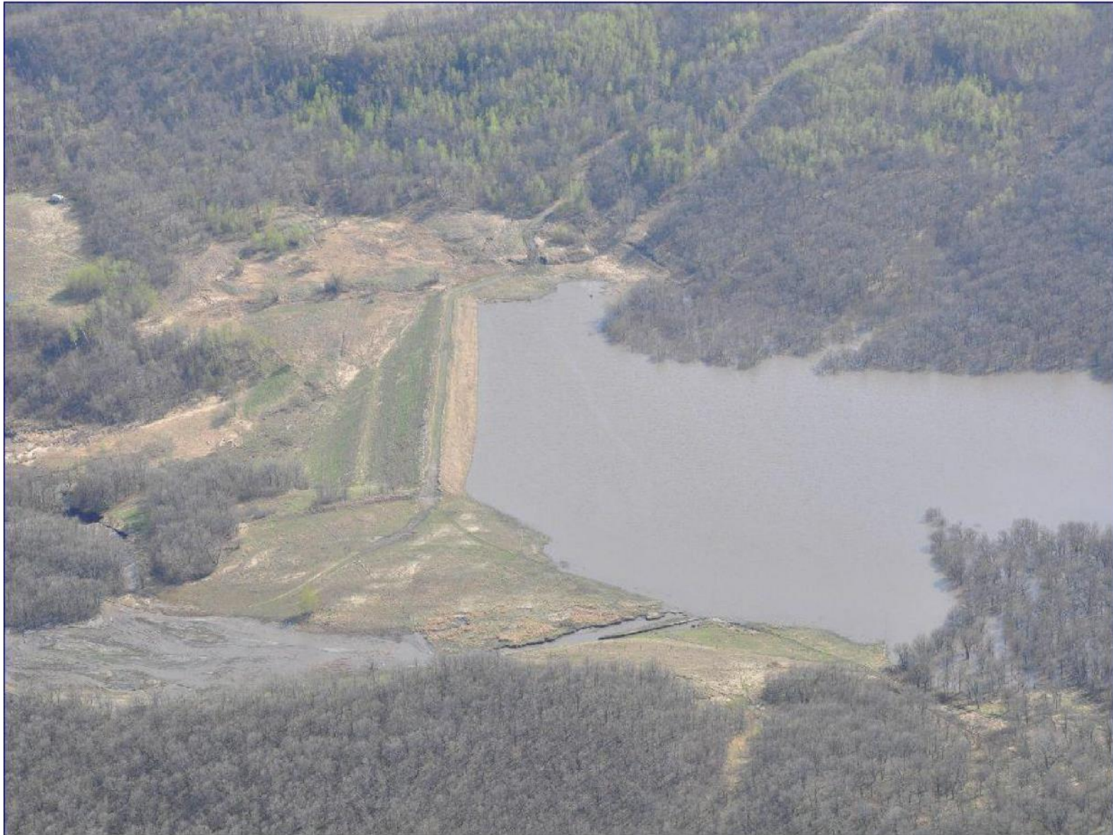
Figure 3.3.2I: 2013 Historic Event Areal Imagery for Bourbanis Dam Looking South
