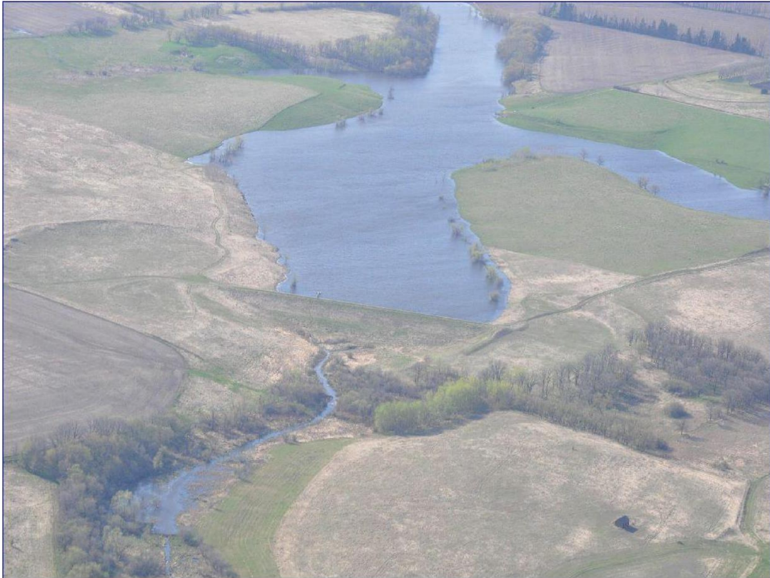
Figure 3.3.2i: 2013 Historic Event Areal Imagery for Weiler Dam Looking Northwest
