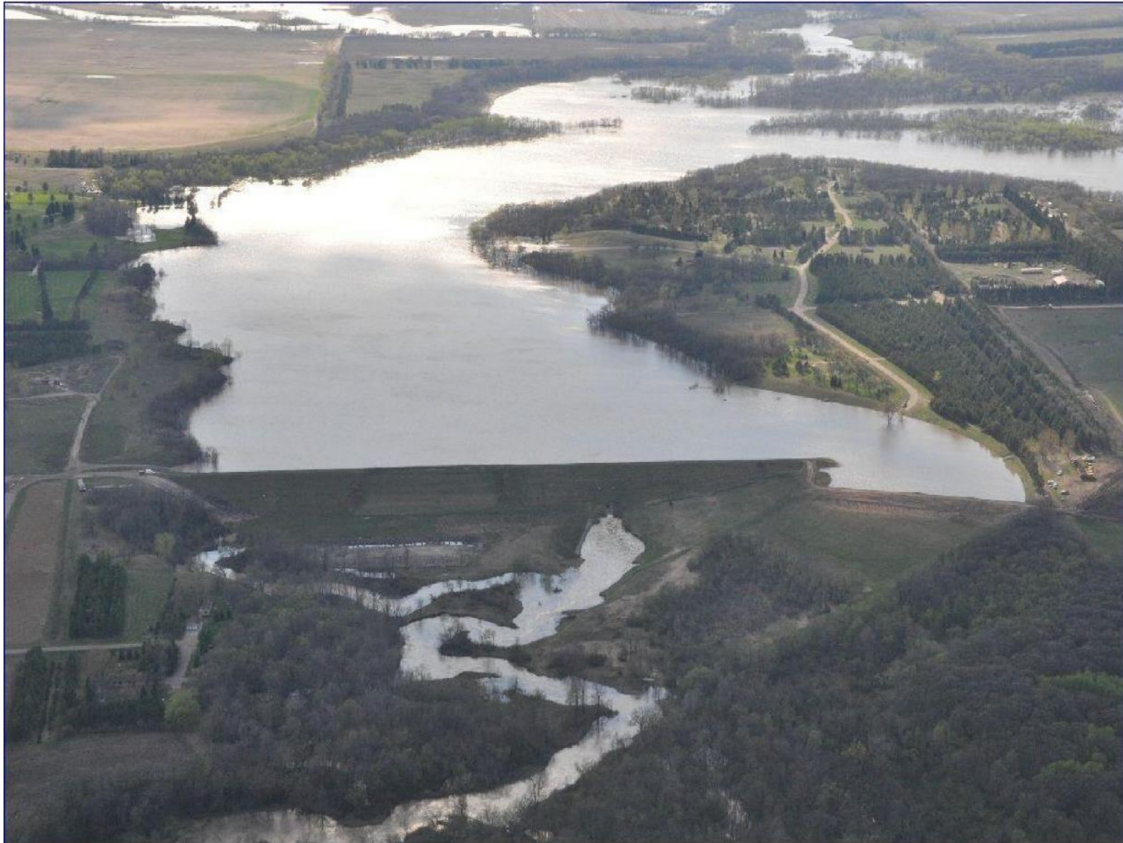
Figure 3.3.2f: 2013 Historic Event Area Imagery for Renwick Dam Looking West
