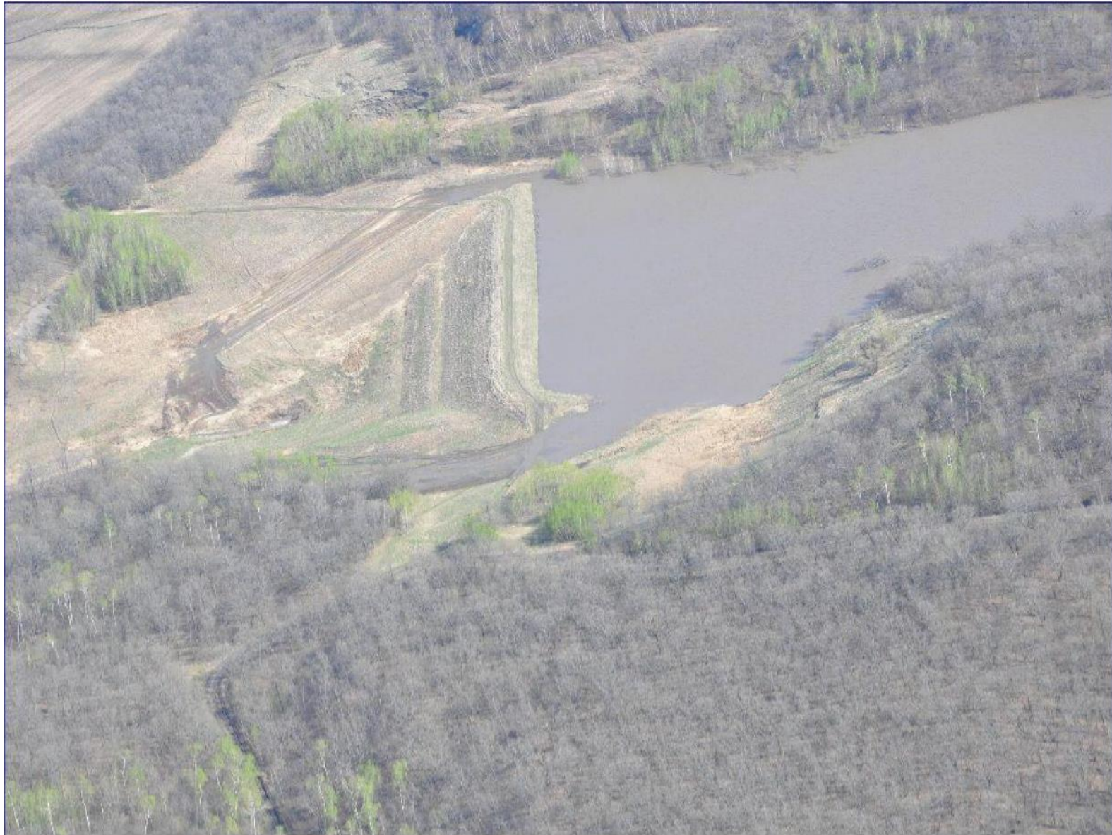
Figure 3.3.2n: 2013 Historic Event Areal Imagery for Olson Dam Looking South
