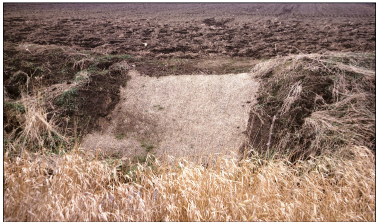
Geotextile reinforced grass chute
