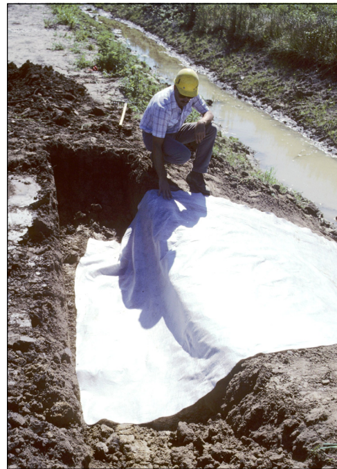
Laying out geotextile for grass chute
