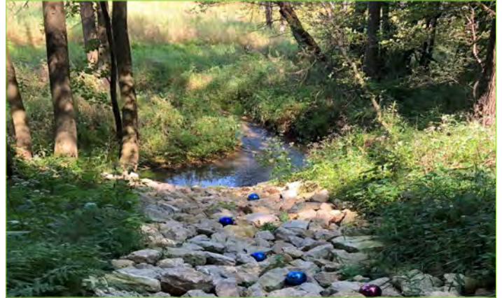
A rock-lined waterway was installed to address gully erosion.
