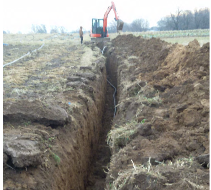
Installing buried pipeline provides for efficient irrigation in the fields and saves on equipment replacement.
