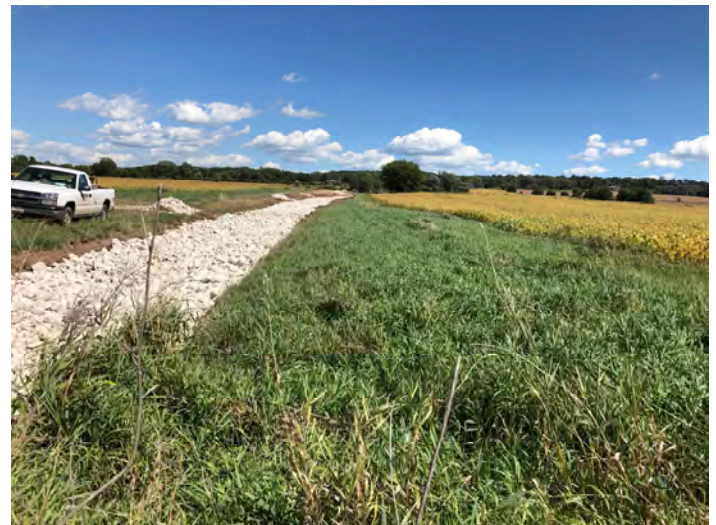
In August 2020, the newly installed, lined waterway with established cover has greatly stabilized the site.
