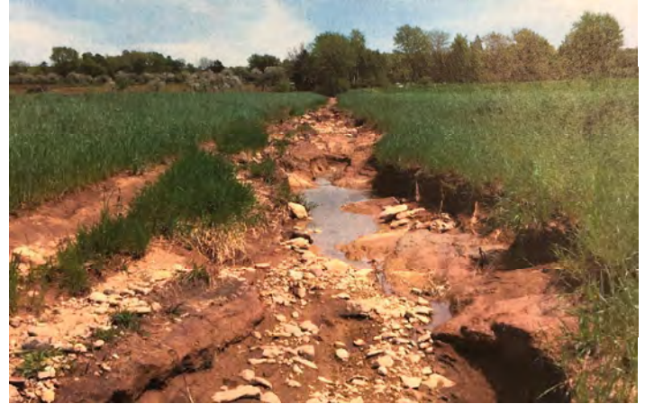
In May 2018, a four-inch rainfall took place overnight, damaging the newly installed grassed waterway.
