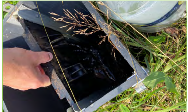
A board is being pulled from the water control structure to lower the water level 6 inches in the upper pond. To raise the water level, more boards can be added.
