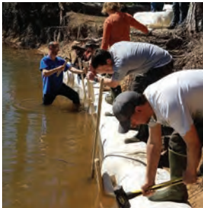
Left: Volunteers and staff work to drive stakes that hold bio-logs in place. Middle: Volunteers and staff work during the second planting event on the streambank. Right: Volunteers and staff work on the streambank stabilization.
