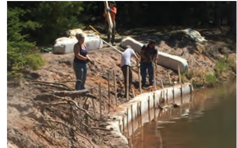
Left: Volunteers and staff work to drive stakes that hold bio-logs in place. Middle: Volunteers and staff work during the second planting event on the streambank. Right: Volunteers and staff work on the streambank stabilization.
