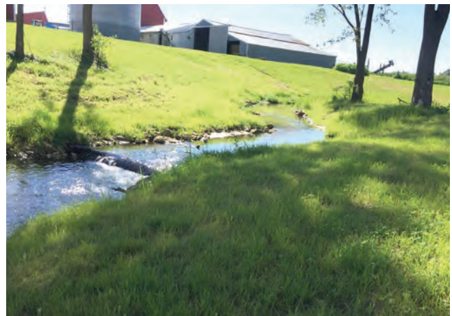
Brion Dairy LLC streambank restoration on Fall Creek.
