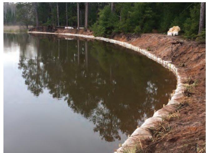
Completed streambank stabilization project.
