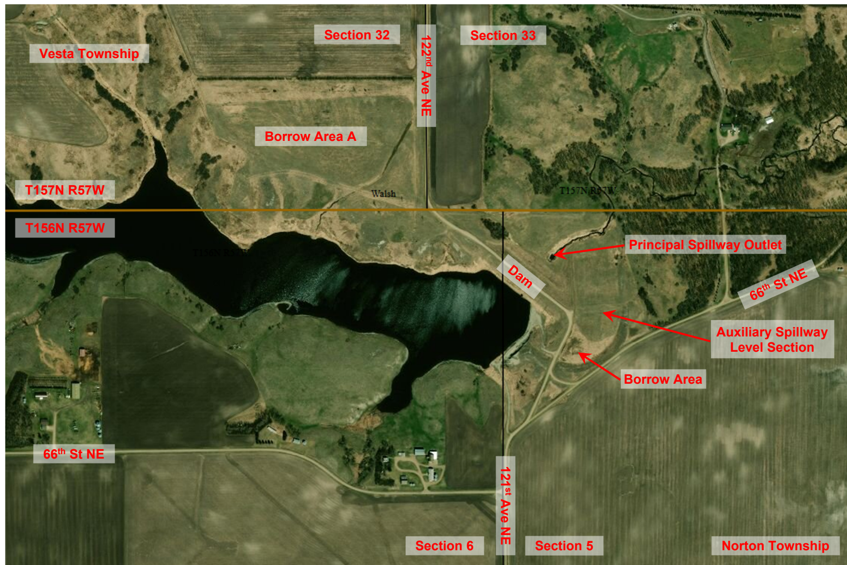
Exhibit 2. Aerial Photo of Bylin Dam (USDA, 2019)
