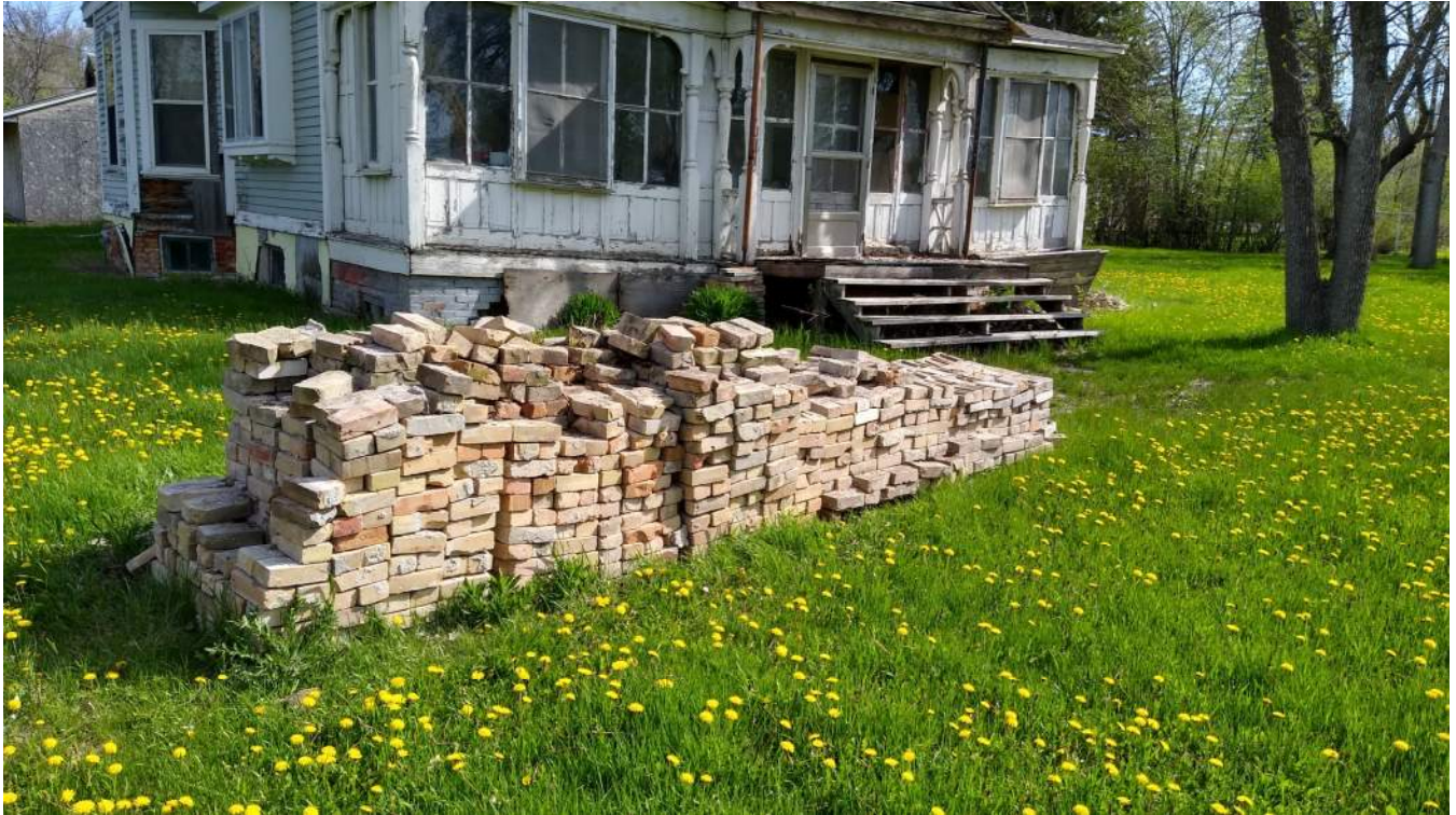
32CS5120 Brick Removal from Structure Foundation
