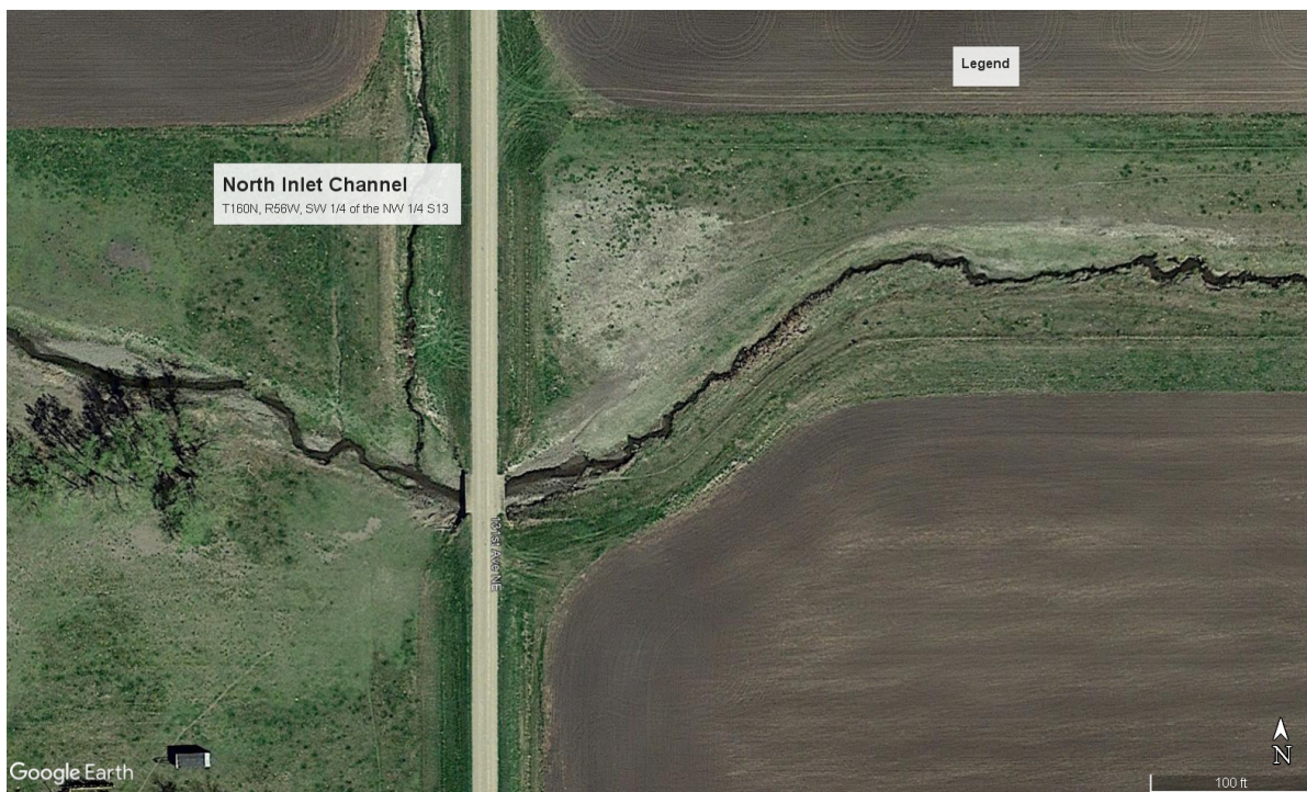
Figure 14: Extant structure at proposed North Inlet Channel. Image: Google Earth 2019
