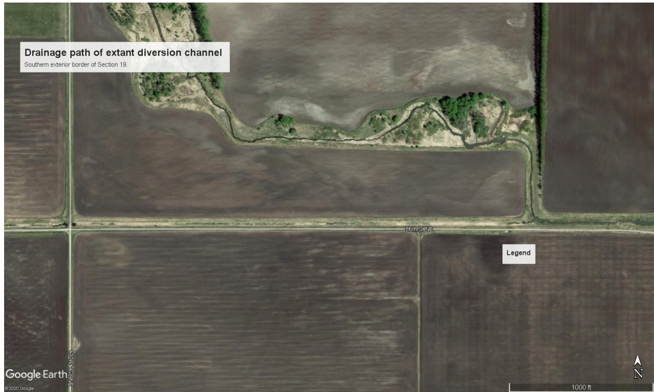
Figure 17: 2019 Satellite view of Section 19 existing drainage improvement. Image Source: Google Earth.
