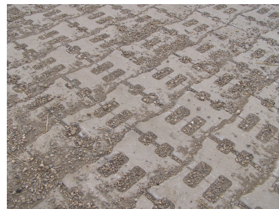
ACBs installed in repair of Lake LaMoire aux. spillway
