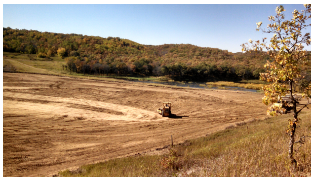
Repair of aux. spillway for Bourbanis Dam in Cavalier County
