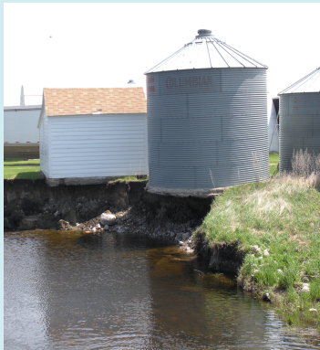
Streambank erosion threatening infrastructure in LaMoure County, ND along Bone Hill Creek
