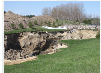
Erosion of aux. spillway at Lake LaMoure
