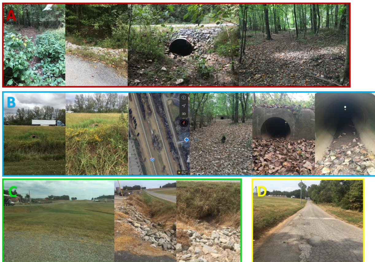
Figure 7: Examples of field trip observations that were used in the hydrological correction process: (A) Ernest Rust road that is heavily wooded with man-made features not clear in satellite images. (B) Series of stops identifying the complex drainage network under I-24. (C) and (D) Field location of false positive drainage points.
