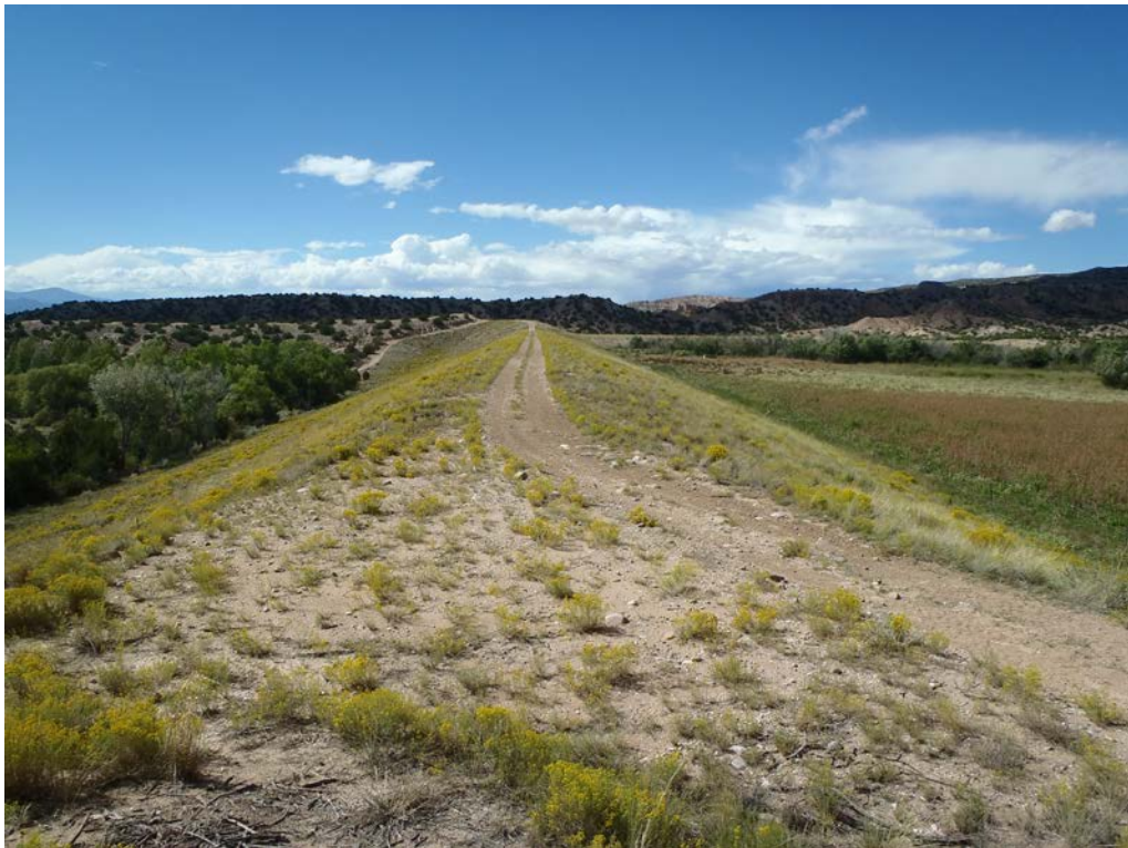
Photograph 2 (9/14/16) – General view of dam embankment looking northwest.
