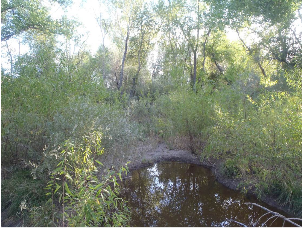
Photograph 21 (9/14/16) – General view of plunge pool and Wetland A at the principal spillway outlet.
