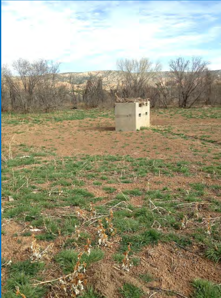
Debris Basin – Sediment Accumulation
