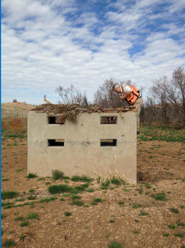
Principal Spillway Riser
