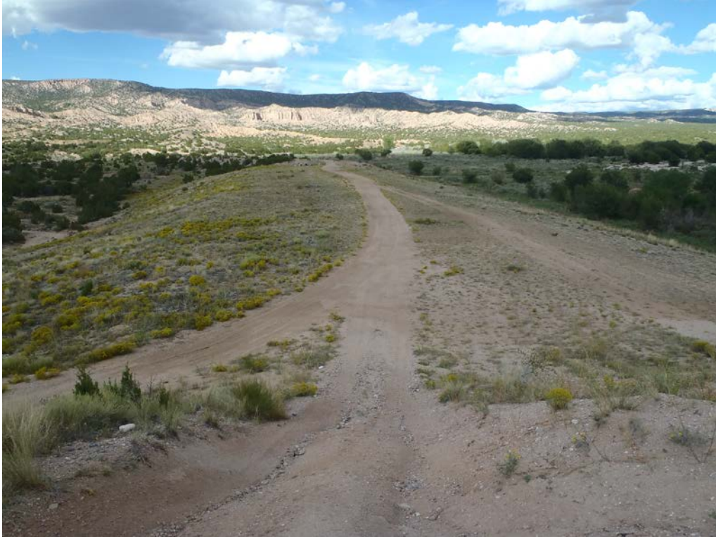
Photograph 3 (9/14/16) – General view of Auxiliary Spillway looking northeast.
