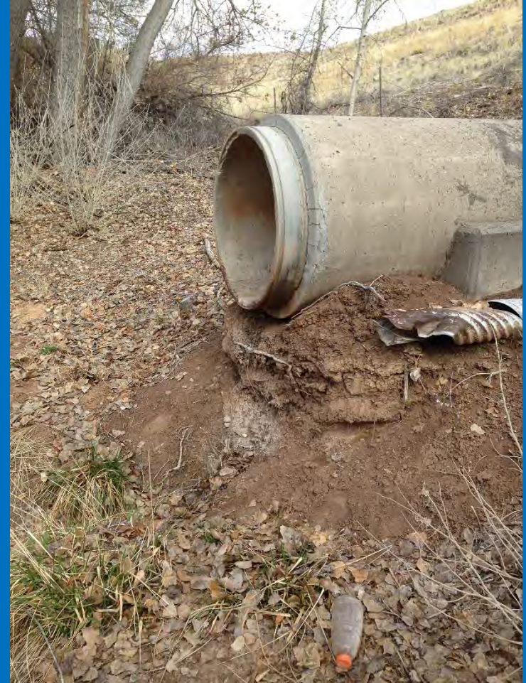
Principal Spillway Outlet Pipe
