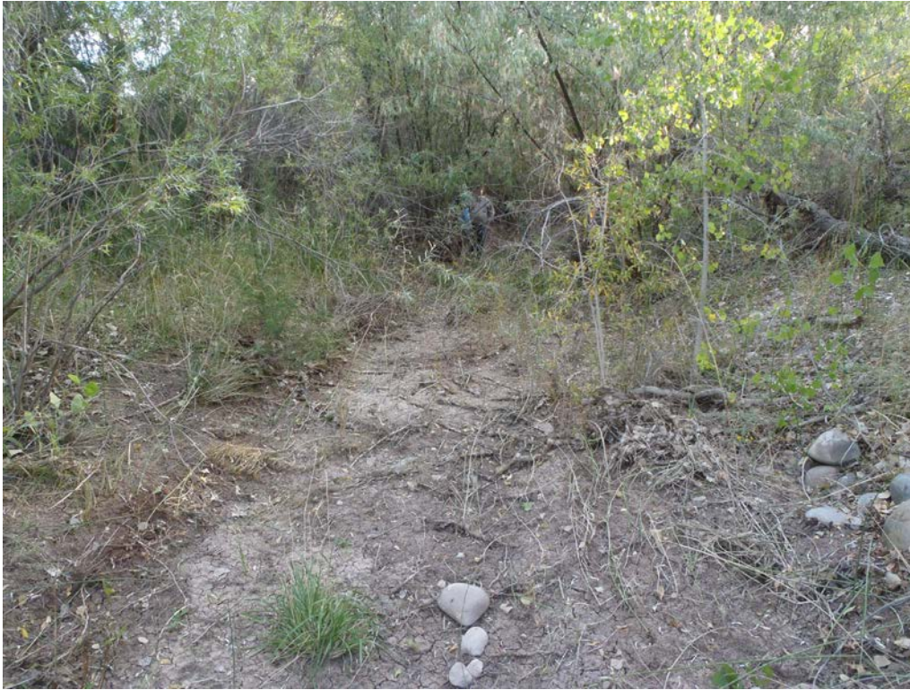
Photograph 7 (9/14/16) – Looking downstream at principal spillway outlet channel for the Arroyo de la Cañada Ancha from plunge pool down to the Acequia de la Cañada Ancha.
