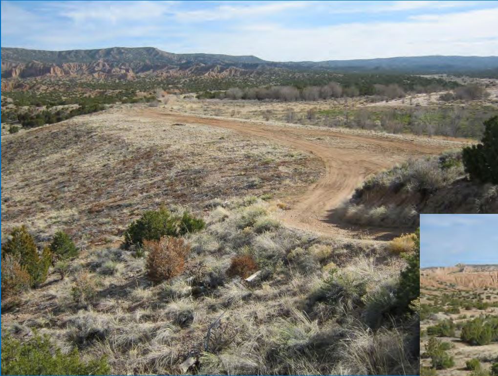
Auxiliary or Emergency Spillway
