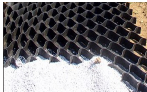
Cellular confinement panels being backfilled with gravel
