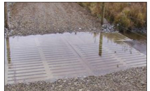
Hog panel stream crossing
