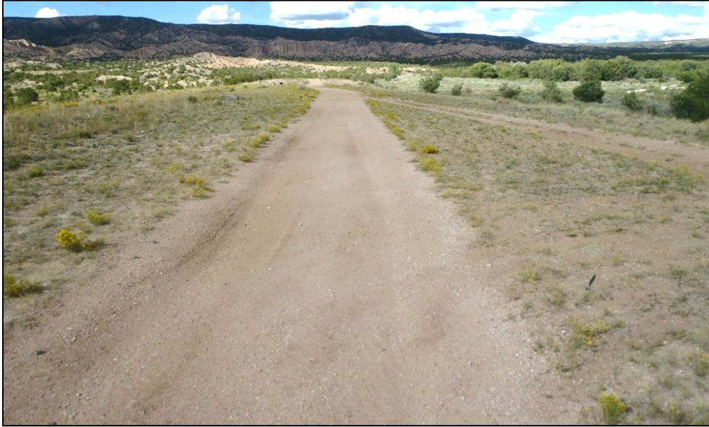
Figure 1-7. Auxiliary Spillway (Looking northeast across the auxiliary spillway)
