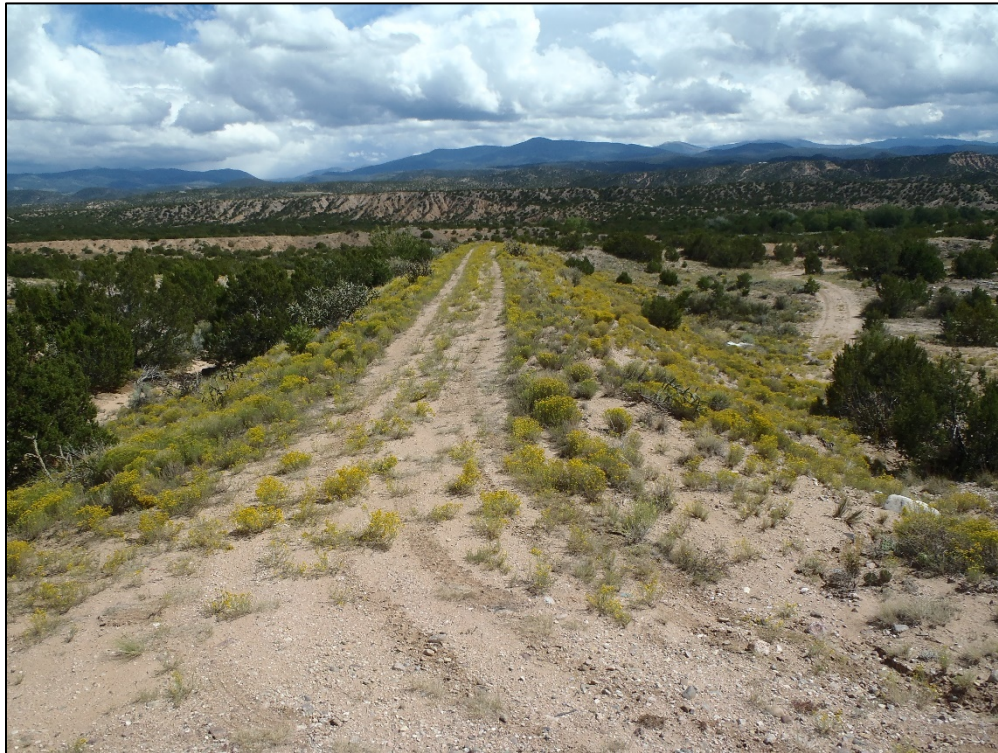
Figure 1-9. Retaining Dike (Looking north across the retaining dike crest)
