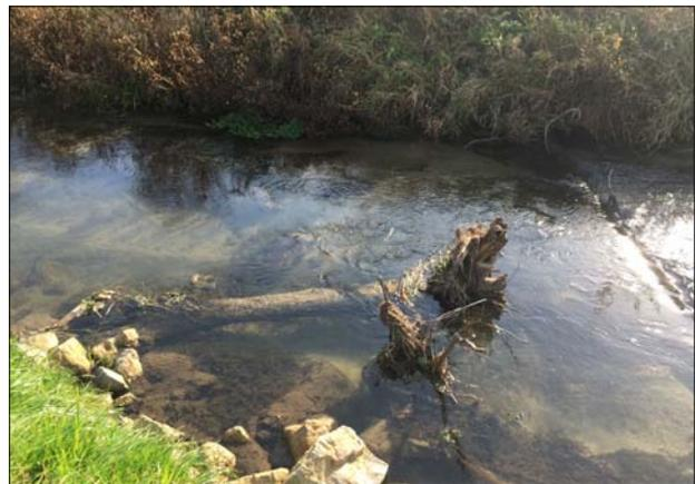
*Spring Coulee Creek after streambank protection and fish habitat installation. Lunker structures, instream wood placement, and in-stream rock placement provide habitat for trout.*
