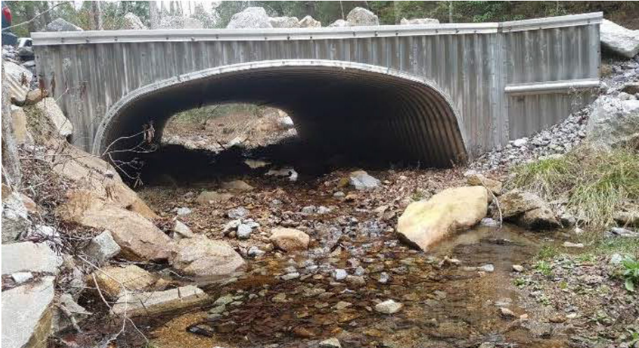
New bottom-less arched culvert with natural stream bed
