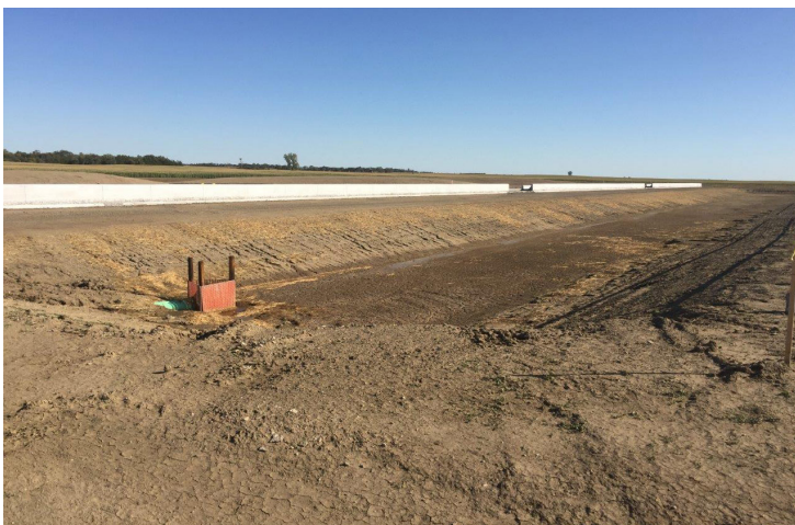
Figure 1. Earthen basin using a hog panel as a screen – passive controlled basin.
