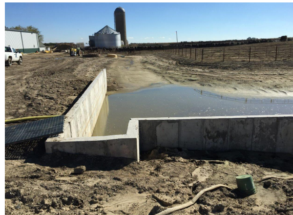
Figure 5. Collection basin with concrete push walls and a picket fence screen mounted in the concrete box outlet.
