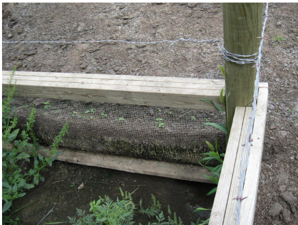
Figure 4. Sediment buildup against a wire mesh filter screen.
