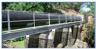
Local sponsors developed the Lower Hamakua Ditch Watershed Project on the island of Hawaii to rebuild and repair a water distribution system that had been built by sugar companies in 1900-1910. The 15 miles of open ditch and 10 miles of tunnel provide irrigation water distribution to 8,000 acres of agricultural lands. This flume replaced an existing one that had deteriorated.
