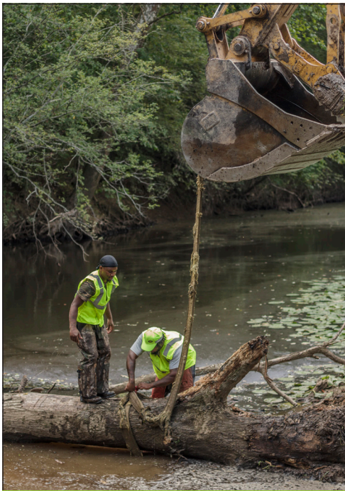
A hand crew clearing and snagging along the Departee Creek channel. Photo by Christopher Willis
