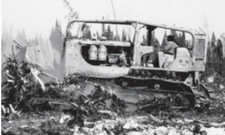
All berms should be placed in straight rows on previously cleared areas (i.e., traction trails) rather than simply be pushed into standing trees and abandoned. This practice greatly improves the burning quality of the berms and cleanup. It also allows farming to proceed between the berms until they can be eliminated. Large berms should be piled as far apart (150 feet or more) as is practical. They are usually burned successfully during the winter.
