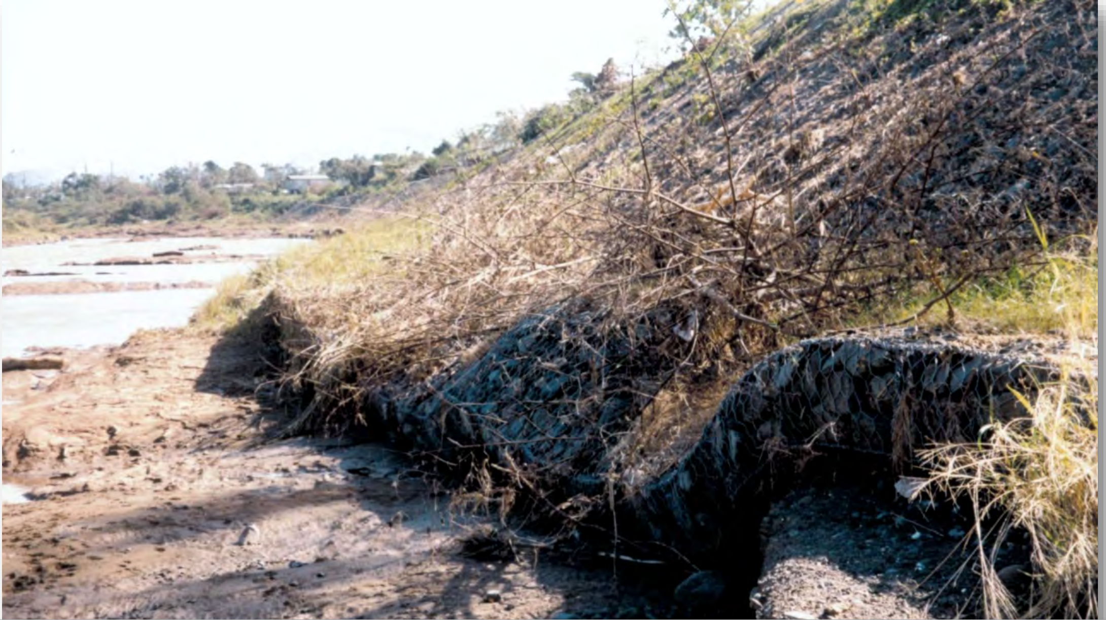
STRUCTURAL MEASURES – GABION MATTRESS
