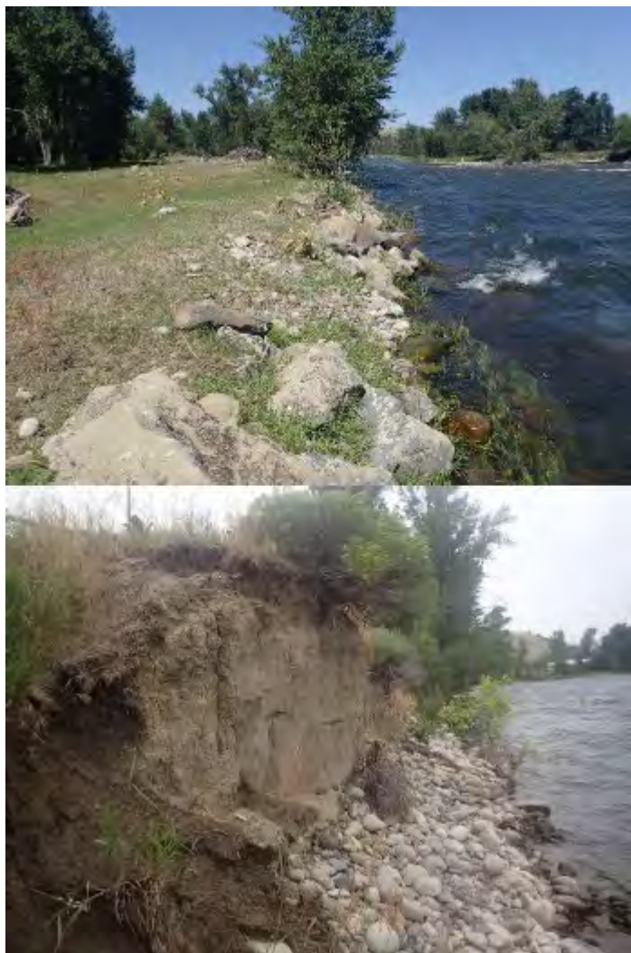
Fig. 19. Top : Overgrazed horse pasture. Notice unmaintained riprap at toe of bank as well as lack of native woody deep-rooted vegetation. Bottom : Riverbank slumping/erosion due to saturation from irrigation water.
