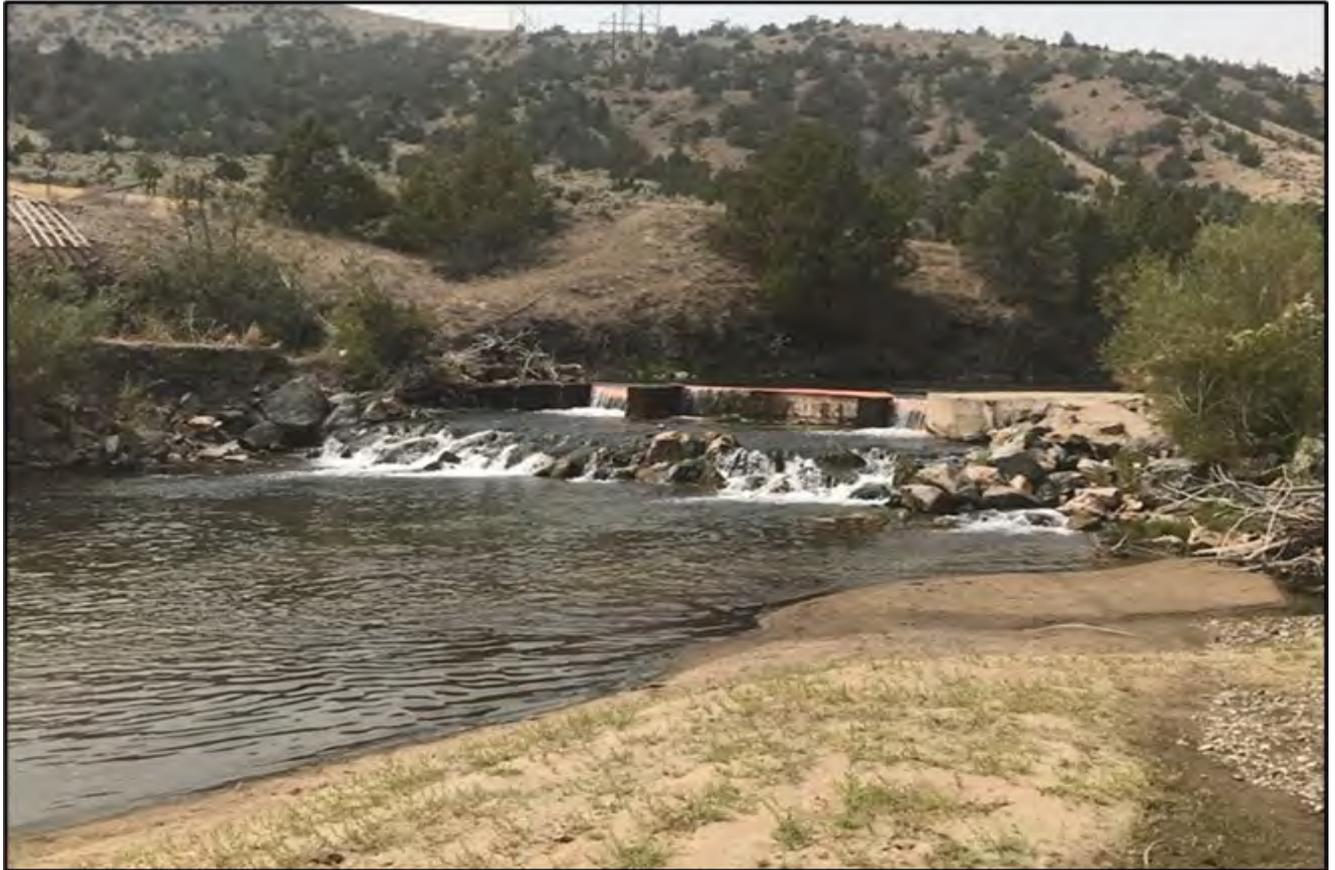
**Figure 3.** Shaw Diversion during irrigation season with flashboards installed. Upstream fish passage is significantly impaired during summer and fall for all fish including adults.
