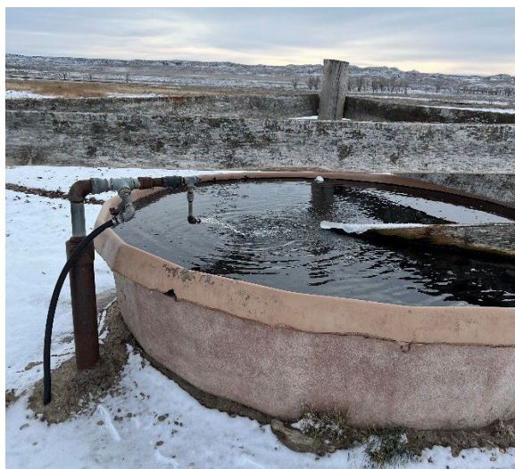
Figure 4 Existing free-flowing artesian well - 20 gpm flow rate
