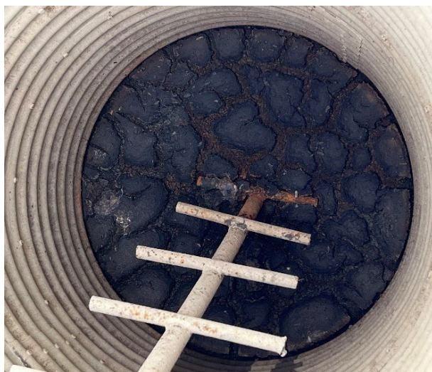
Figure 3: Sediment accumulated inside the culvert.
