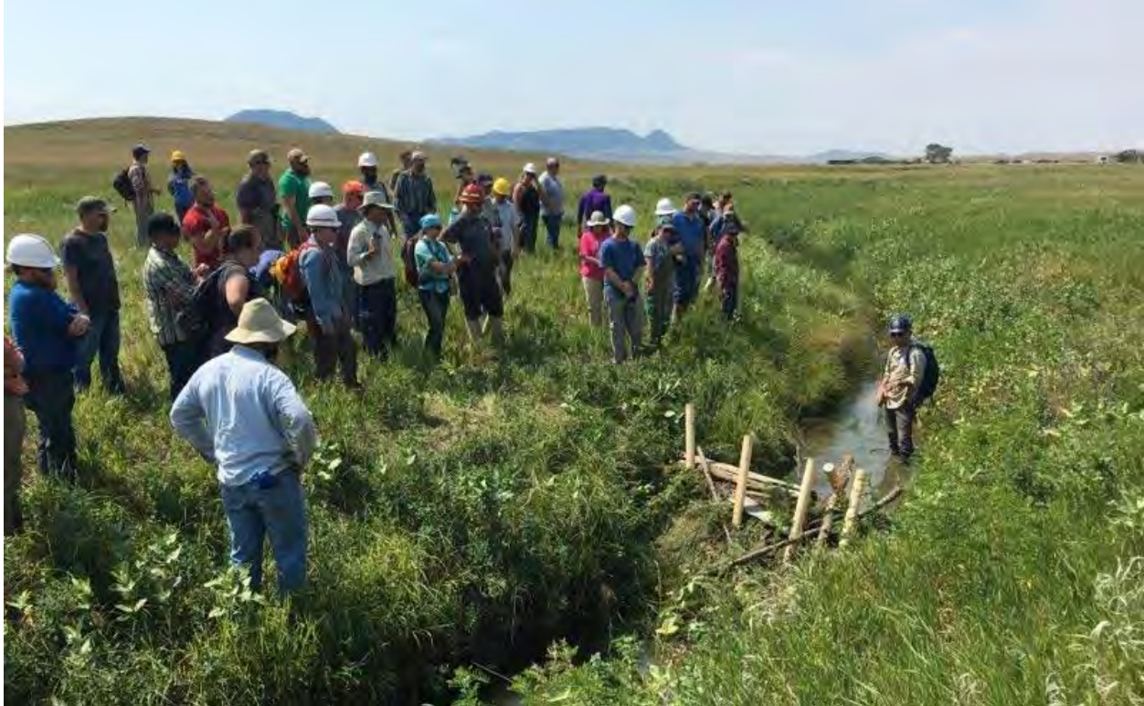
Installation of BDAs during 2019 workshop on Bear Creek.
