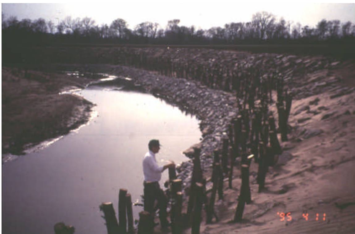
Figure 7.9 Longitudinal Peaked Stone Toe Protection In Combination With Willow Post Upper Bank Protection
