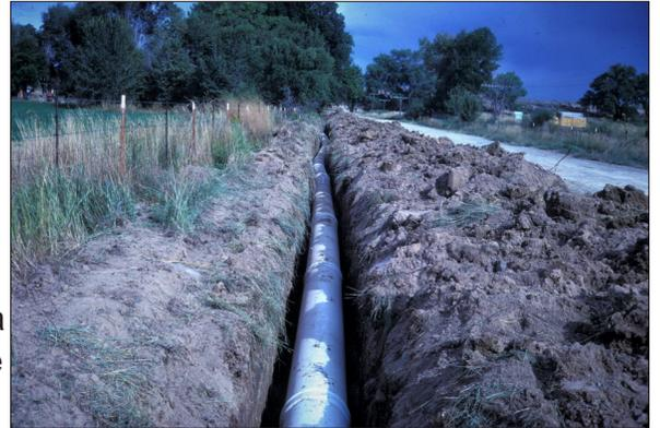
An irrigation pipeline can be made of flexible conduit materials, such as plastic, steel, aluminum, corrugated metal, or ductile iron pipe, or it can be made from rigid conduit, such as concrete or plastic mortar pipe. The pipeline can be installed underground or above ground.
