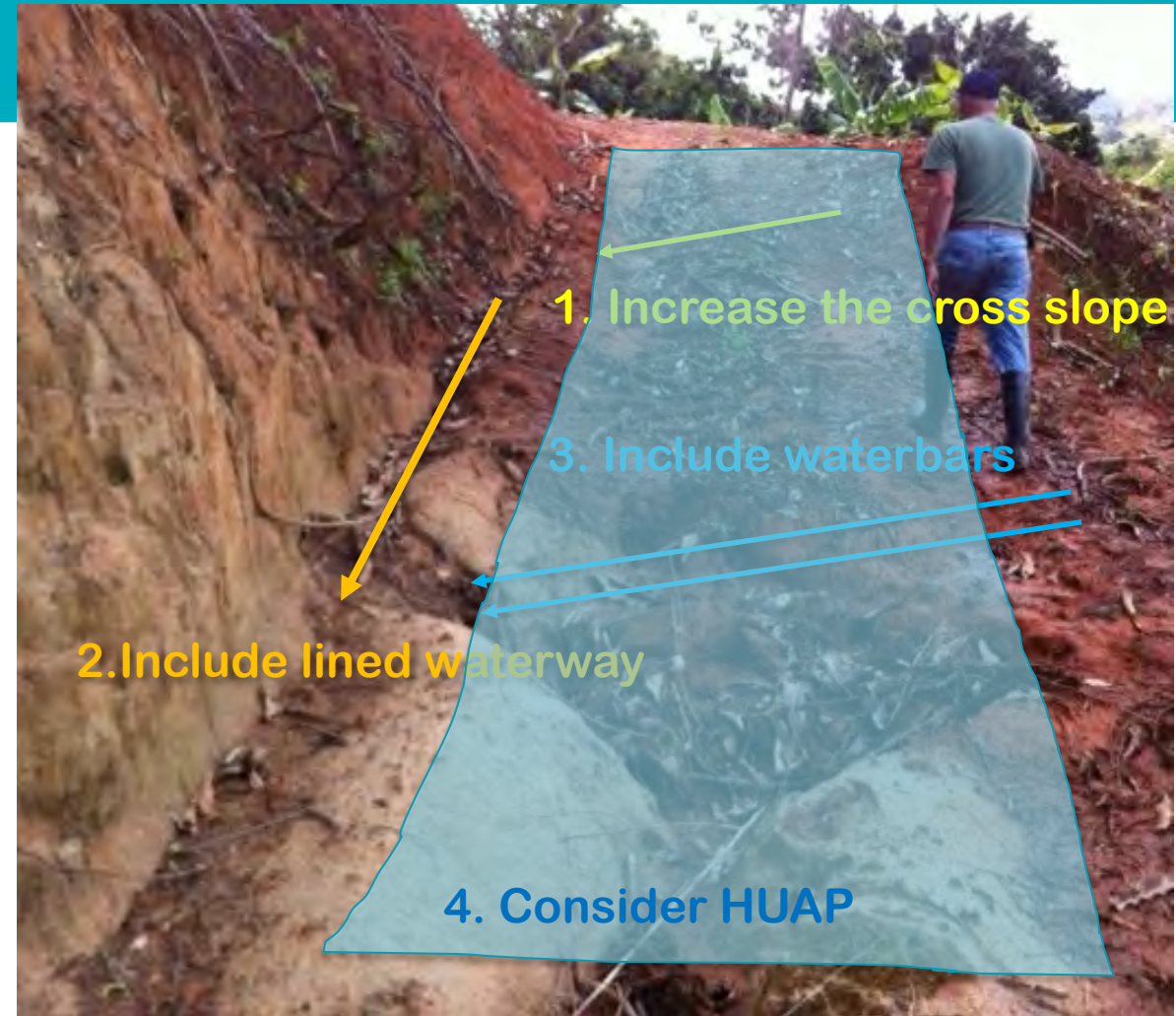
Figures 41& 42 : HUAP, concrete or crusher run (mogolla) w/ geotextile recommended only on the steepest and worst areas. Jayuya, PR.
