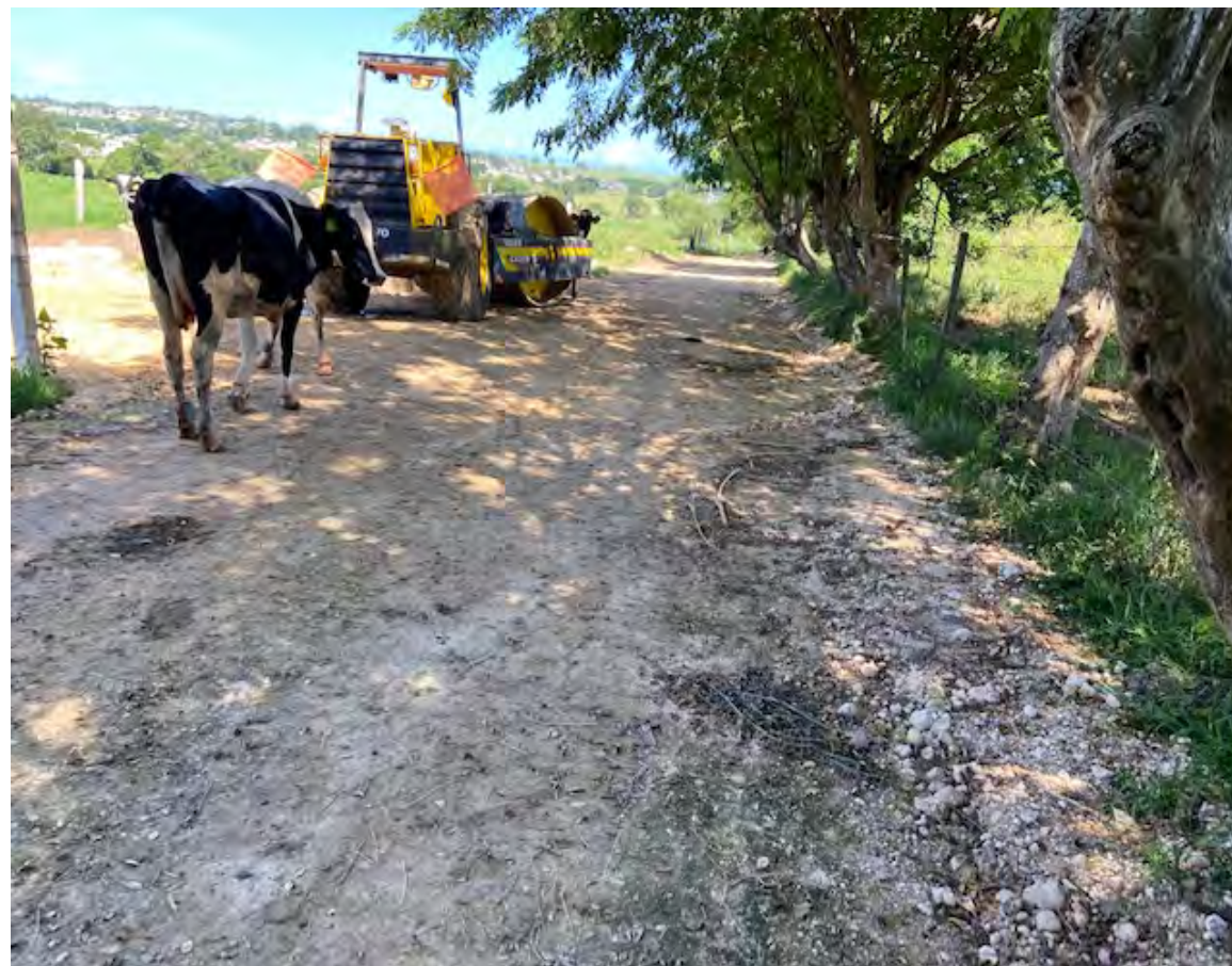
Figure 18: Aggregate compacted with roller.
