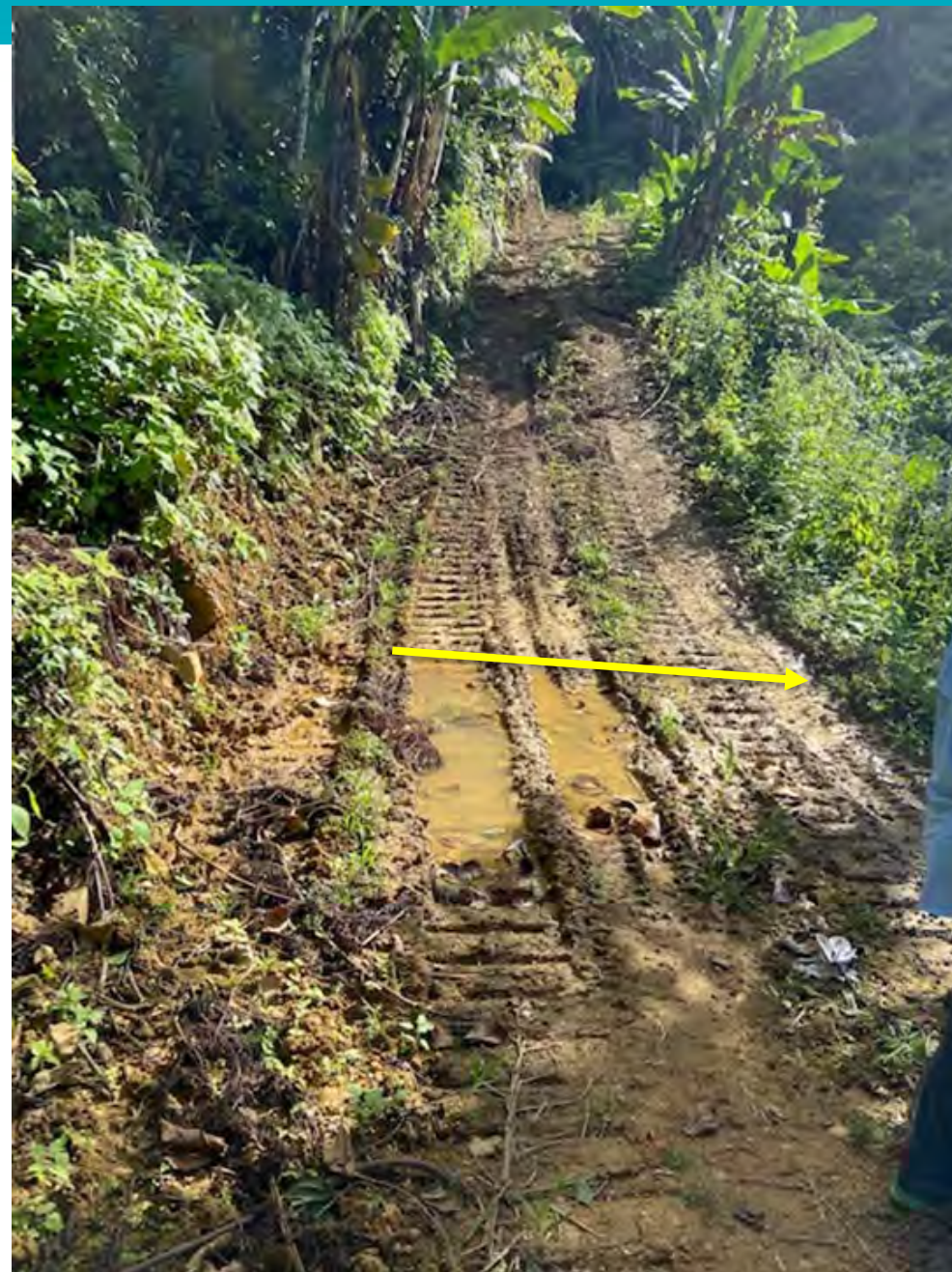
Figure 8: HUAP, concrete or crusher run aggregate (mogolla)w/ geotextile recommended. Jayuya, PR.
