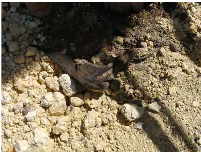
Figure 22: Geotextile bellow aggregate
