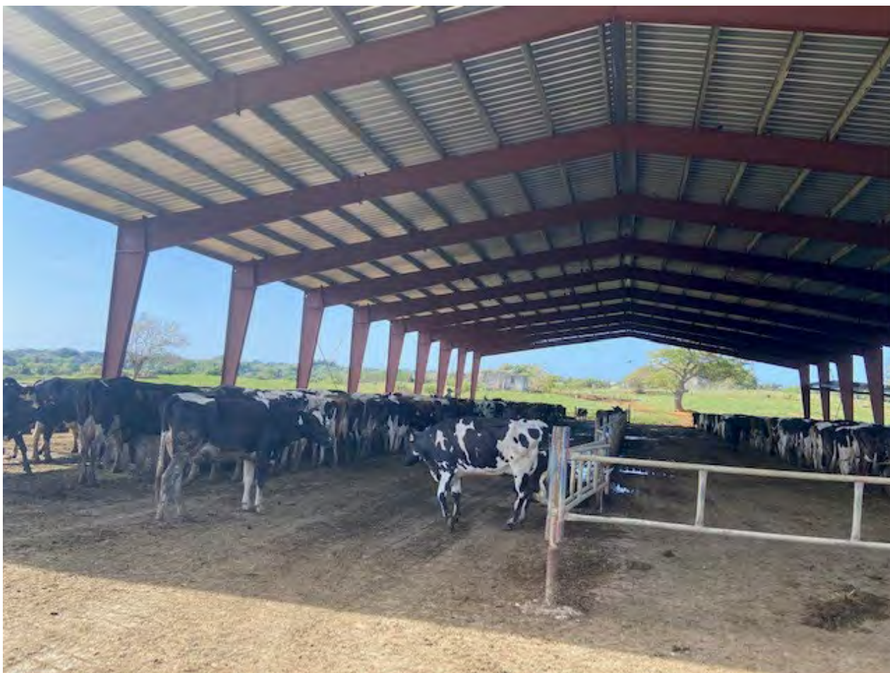
Figure 5: HUAP, concrete, inside a feeding area. Hatillo, PR.
