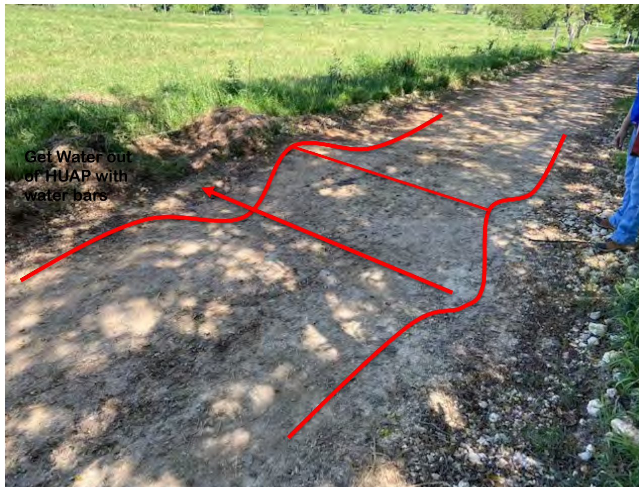
Figure 19: Water bar formed with aggregate and compacted with roller.
