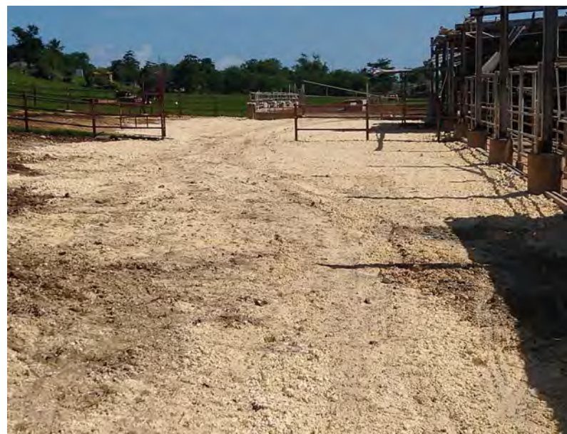
Figures 23 & 24: Installed HUAP with geotextile and aggregate.
