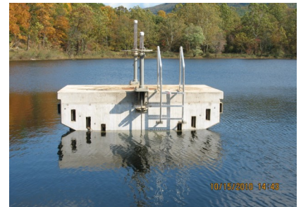
Above: Existing riser at Huntsman Lake. Below: Example of closed top riser.
