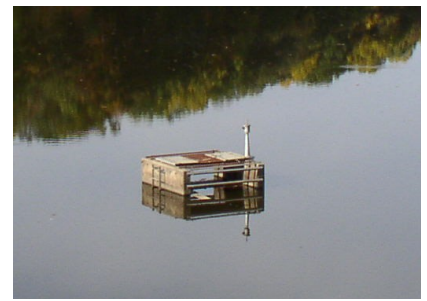
Above: Existing riser at Huntsman Lake. Below: Example of closed top riser.
