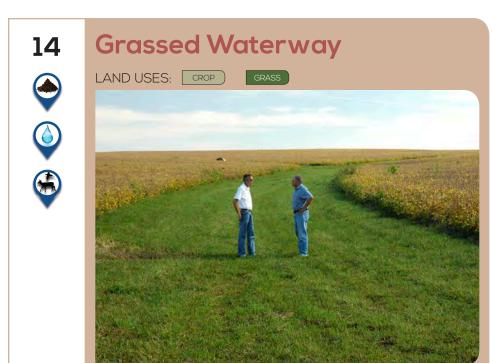
Grassed waterways are shaped constructed channels that are seeded to grass or other suitable vegetation to convey water to a stable outlet at a non-erosive velocity.
