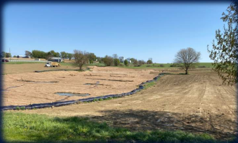
Sediment removal and construction
