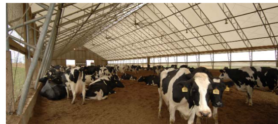
Figure 2.3 A hybrid-ventilation dairy barn.
