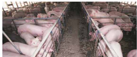
Figure 2.2 A mechanically-ventilated swine finishing barn.
