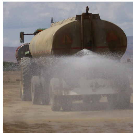
Figure 6.5 Water application to an unpaved surface.
