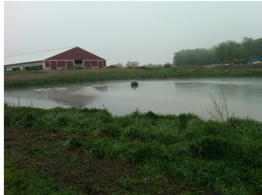
Figure 3.5 Aerobic circulator on a dairy lagoon.
