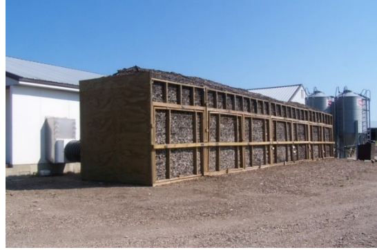
Figure 2.8 A vertical bed biofilter at a University of Minnesota research farm (image courtesy of Iowa State University).
