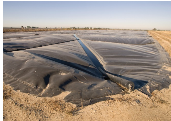
Figure 3.7 Covered lagoon anaerobic digestion in California.
