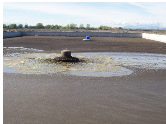
Figure 3.4 Mechanical aeration of a manure storage.
