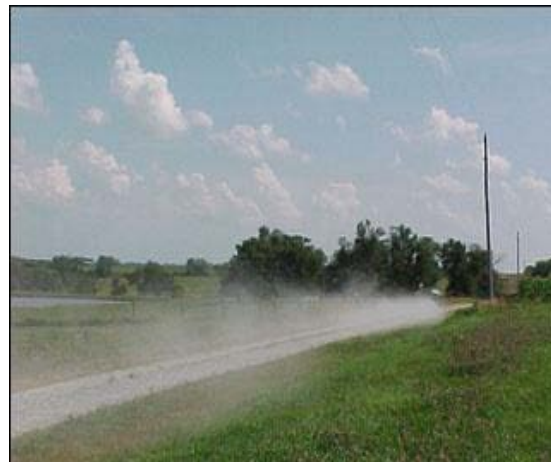
Figure 6.3 Dust from unpaved roadways.
