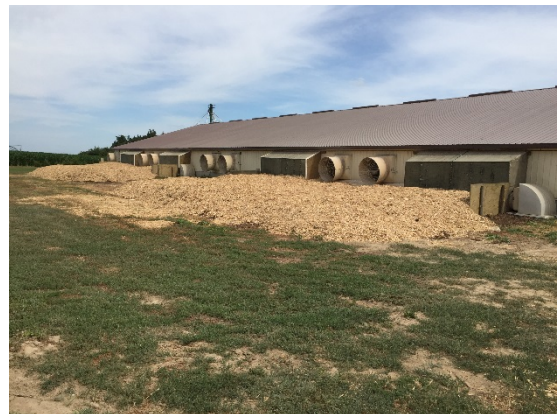
Figure 2.7 A flat open bed biofilter.
