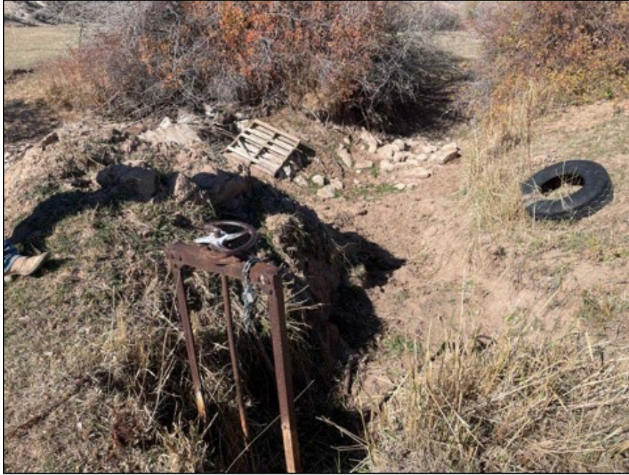
Photo 12: The Buck Diversion on Woodruff Creek. The diversion was dry at the time of survey. Human-made debris is present in the creek bed and irrigation canal.
