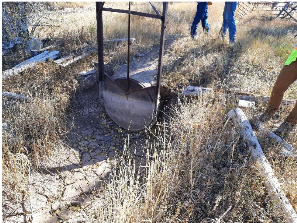
SC107 Typical Site Conditions | East
