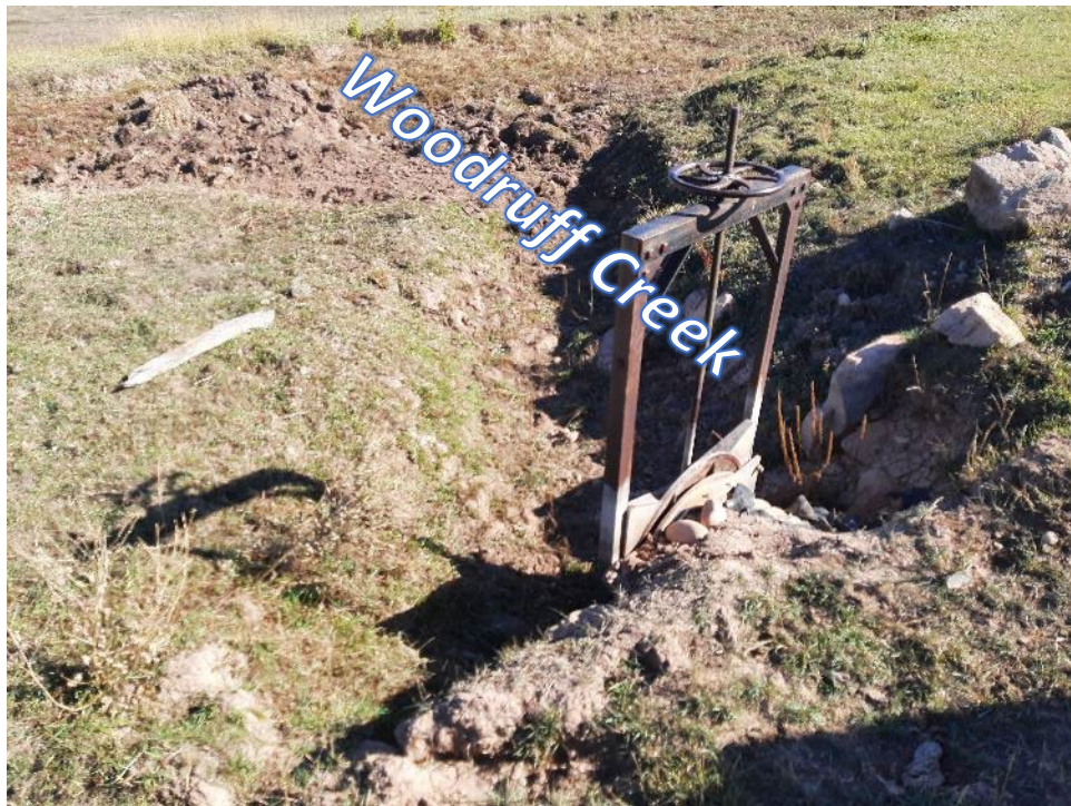
SC103 Typical Site Conditions | North
