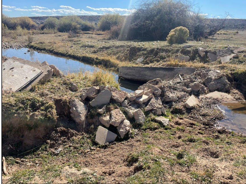
Photo 14: The Hagus Diversion on Woodruff Creek. Riprap and concrete has been used to construct the diversion.
