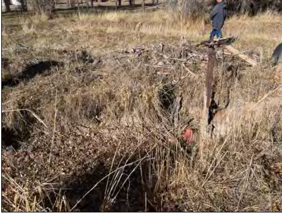
Photo 10: The Tingey/Byson/Eastman Diversion on Woodruff Creek lies in a residential area in Woodruff. The canal adjacent to this diversion is dry. Human made debris is present in the canal.
