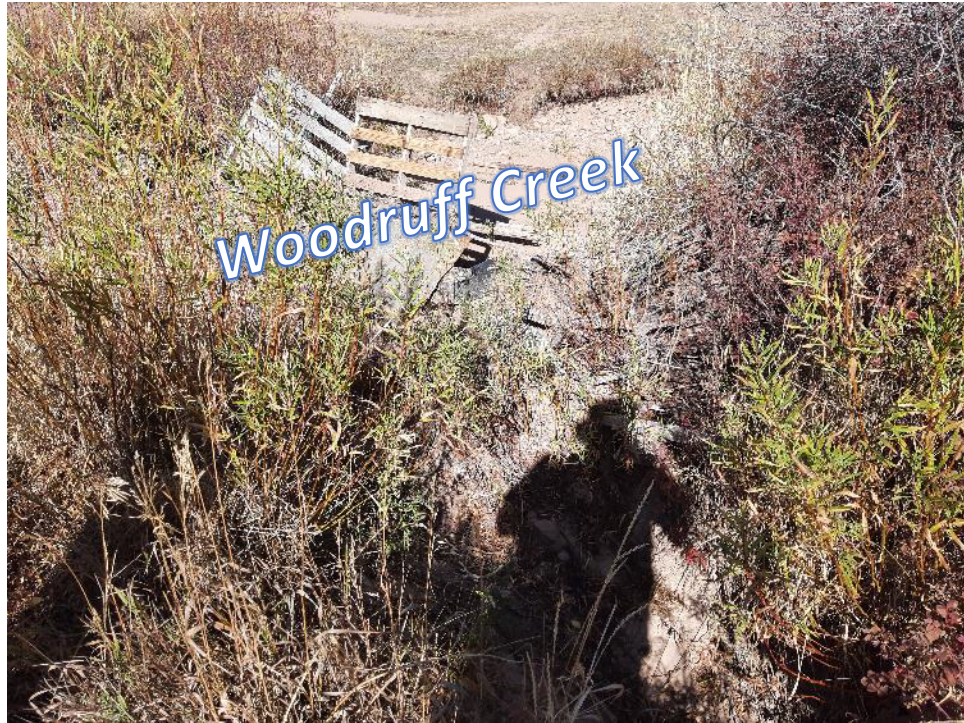
SC106 Typical Site Conditions | West
