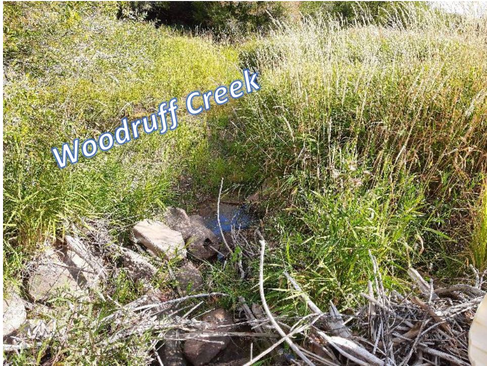
SC18 Typical Site Conditions | North
