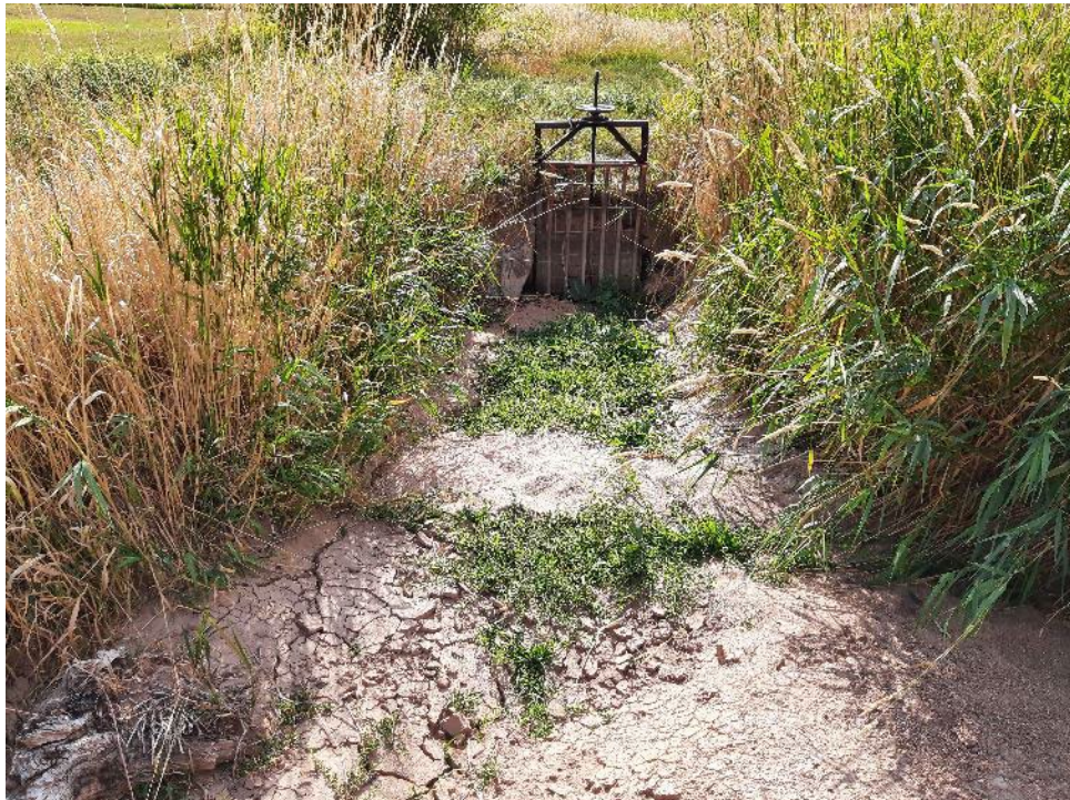
SC17 Typical Site Conditions | East
