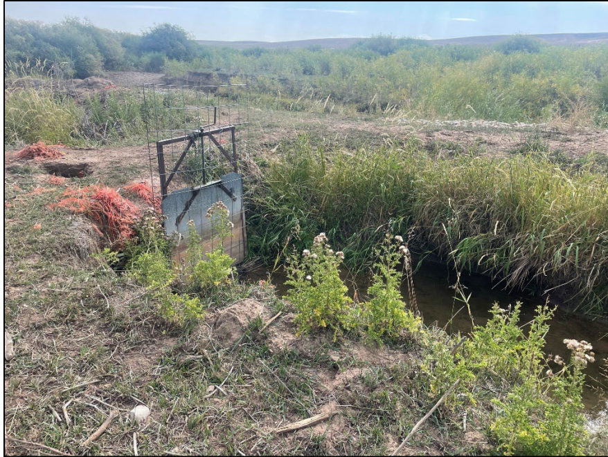
Photo 7: Frazier #1 Diversion on Woodruff Creek. Bailing twine debris is present around and in the diversion.
