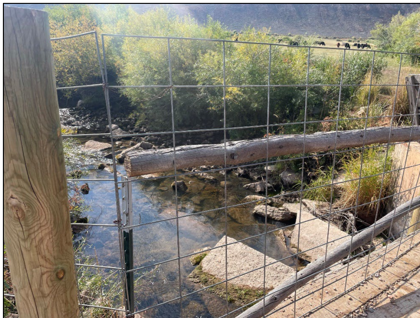
Photo 5: Eastman/Frazier Diversion on Woodruff Creek.
