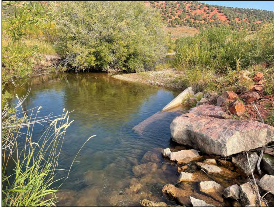
Photo 4: Riprap and concrete have been placed in Birch Creek at the Putnam/Cornia Diversion.
