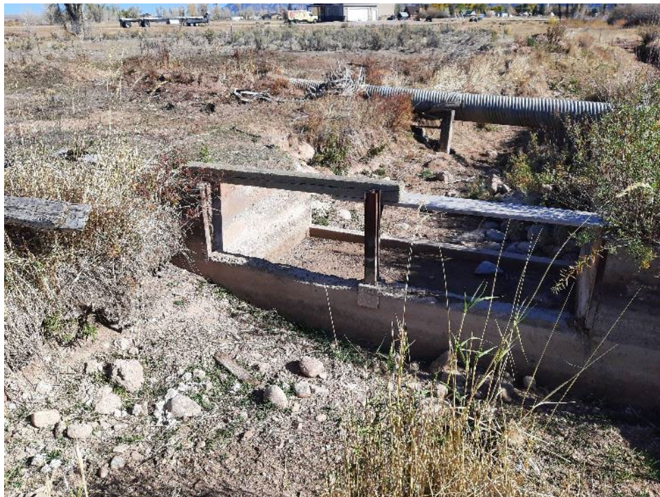
SC105 Typical Site Conditions | North
