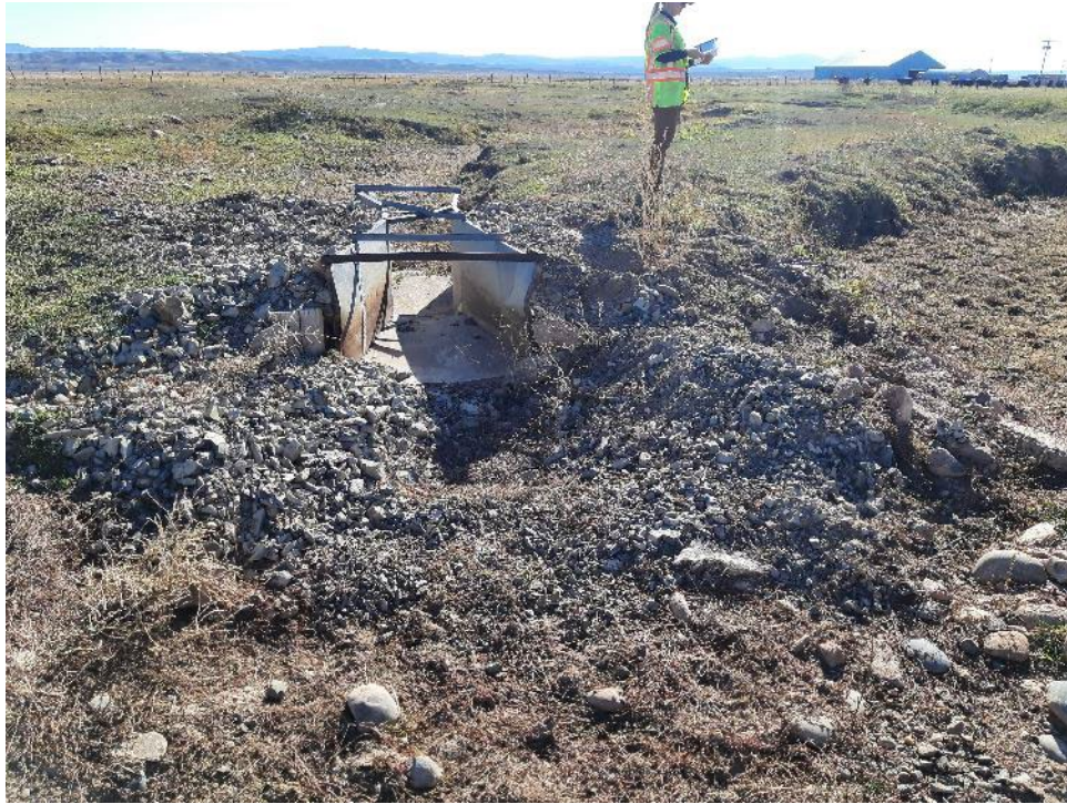
SC104 Typical Site Conditions | East
