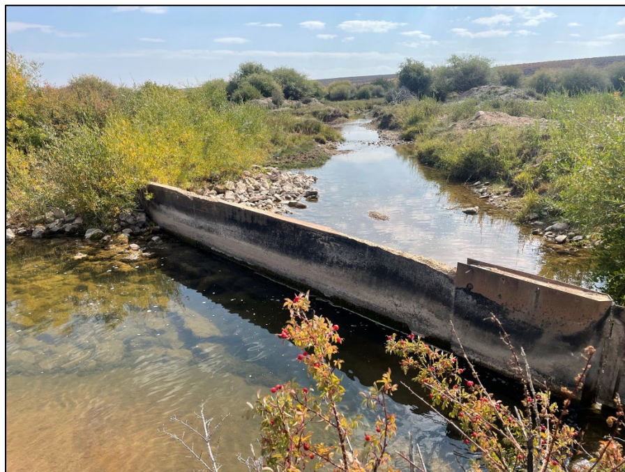
Photo 9: The Splitter Diversion on Woodruff Creek. A cement barrier is constructed as part of the diversion structure. Riprap and a metal walkway are present (not pictured).
