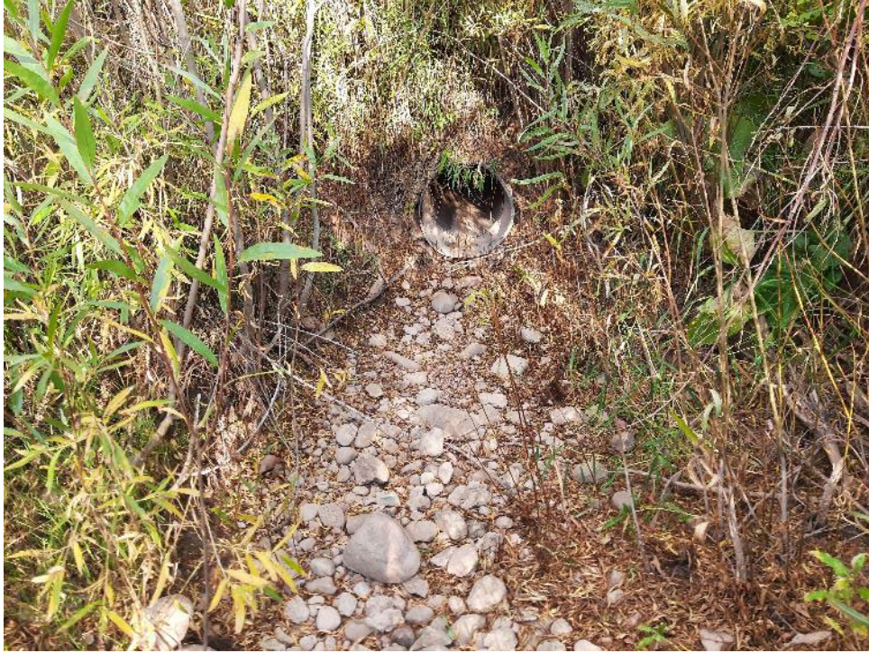
SC08 Typical Site Conditions | West
