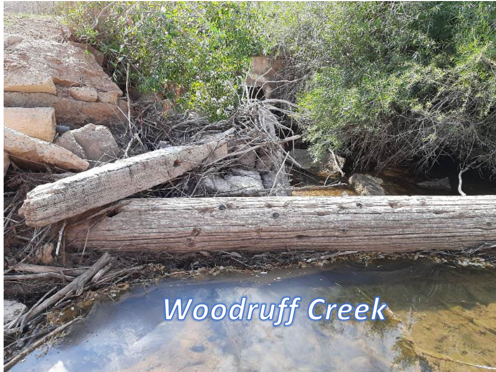
SC16 Typical Site Conditions | East
