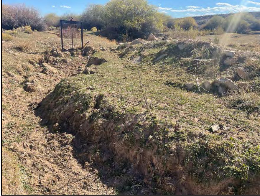
Photo 15: Soil has been filled into the connected canal at the Hagus Diversion on Woodruff Creek.
