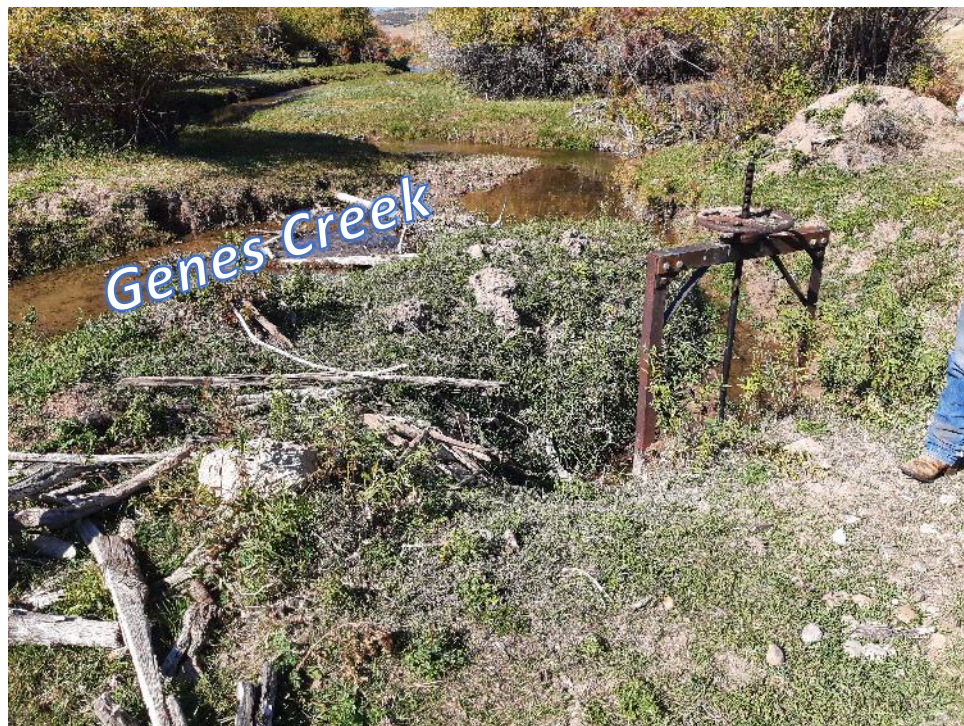
SC109 Typical Site Conditions | West
