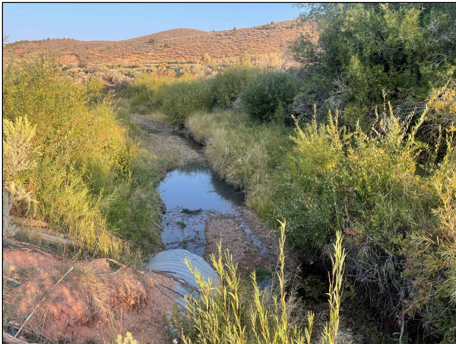
Photo 2: Birch Creek at the Smith Ditch Diversion.
