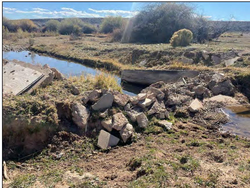
Photo 14: The Hagus Diversion on Woodruff Creek. Riprap and concrete have been used to construct the diversion.
