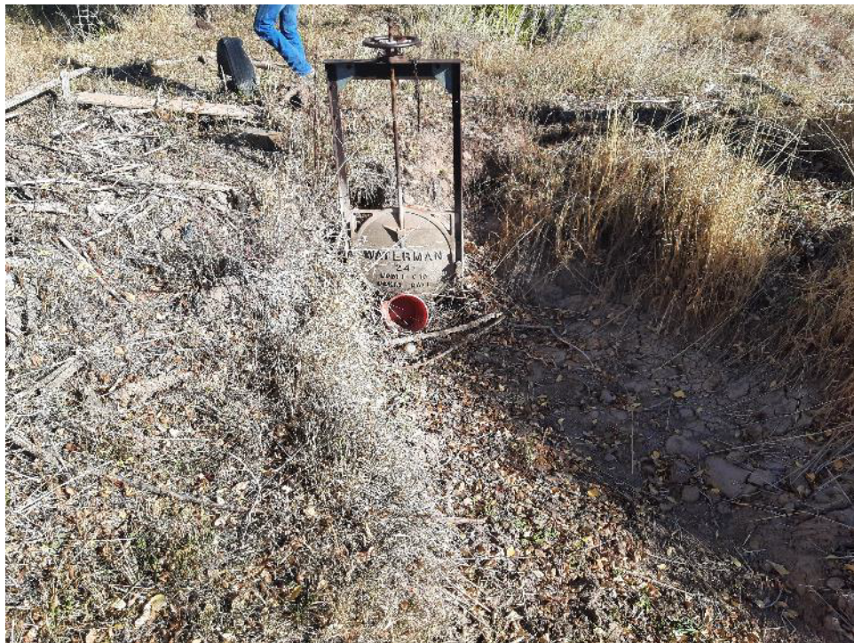
SC101 Typical Site Conditions | North
