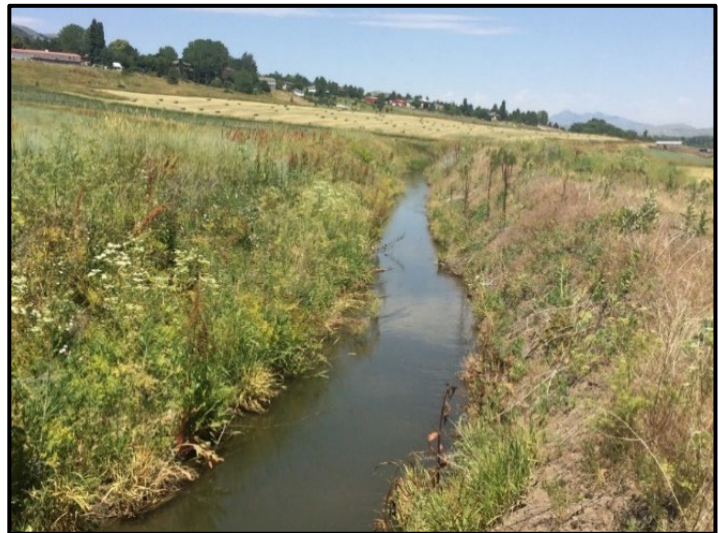
Figure 2-7: Earthen Segment of the Lower Canal
