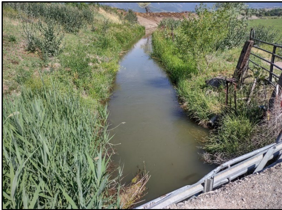
Figure 2-8: Wellsville East Field Canal
