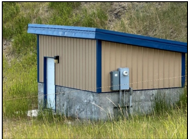
Figure 3-7: Arsenic Contaminated Well Near Project Area
