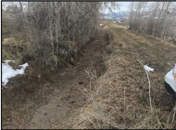
Figure 2-6: Earthen Segment of the Upper Canal
