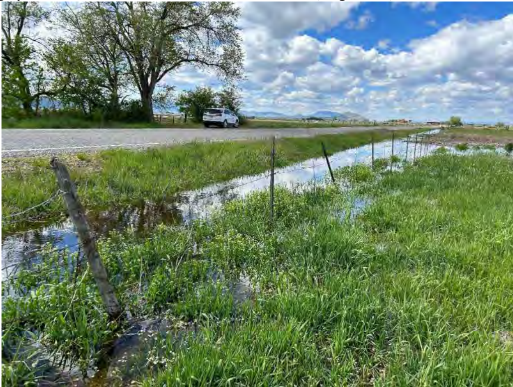
Photograph 17: Northern view of flooded ditch 70 and wetland 20 between road prism and pastureland.
