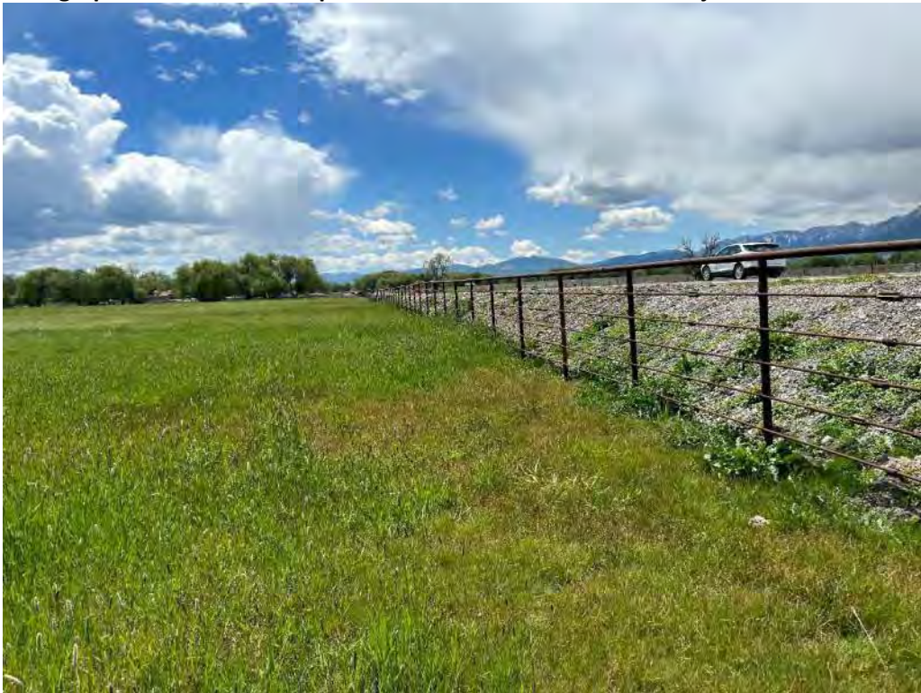
Photograph 27: South view of upland pastureland with newly constructed road prism.
