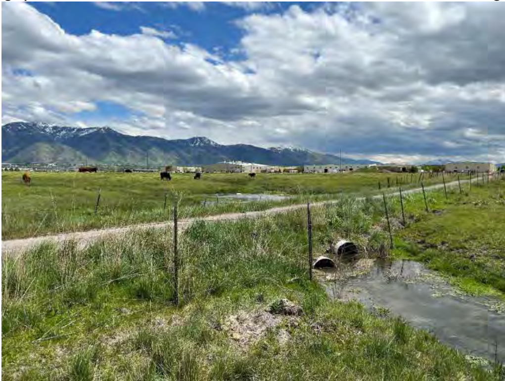
Photograph 22: Southeastern view of wetland 4 and culverts under road prism.
