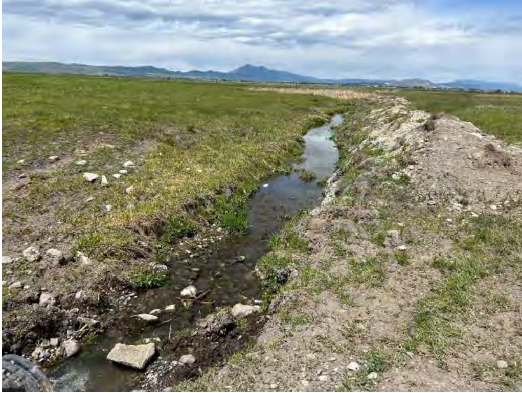
Photograph 21: Northwestern view of culvert outflow with ditch 38 and disturbed bare ground.
