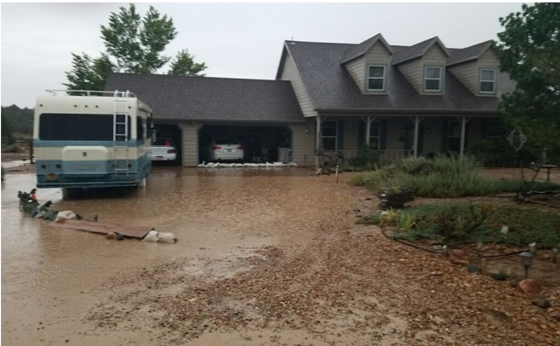
Photograph C-2. Flooding in Dammeron Valley, Utah.
