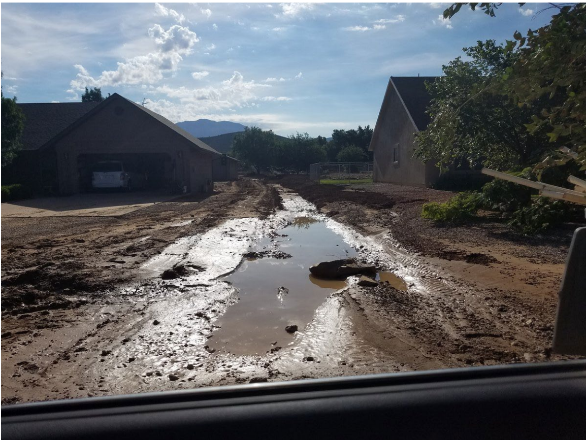
Photograph C-5. Flooding in Dammeron Valley, Utah.
